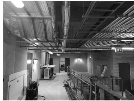
Image 2 Practice-based case study - Main mechanical and electrical services routes
