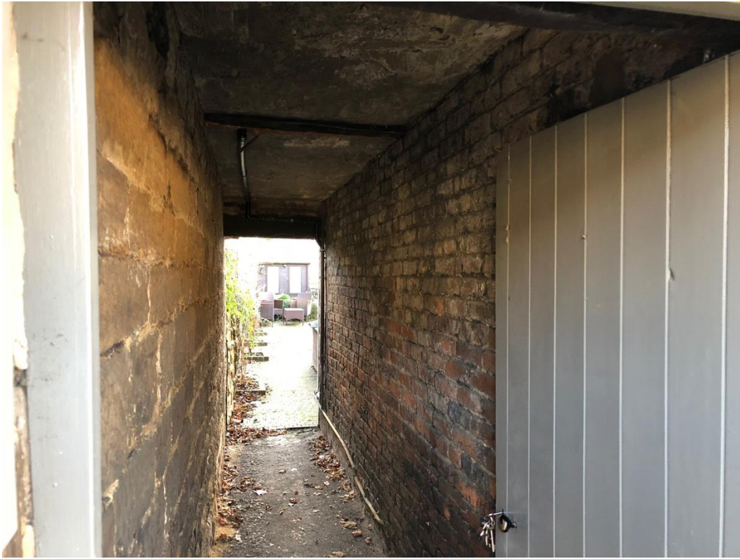
Image 3. Passageway underneath the property. The main bedroom sits partly over this passageway.
