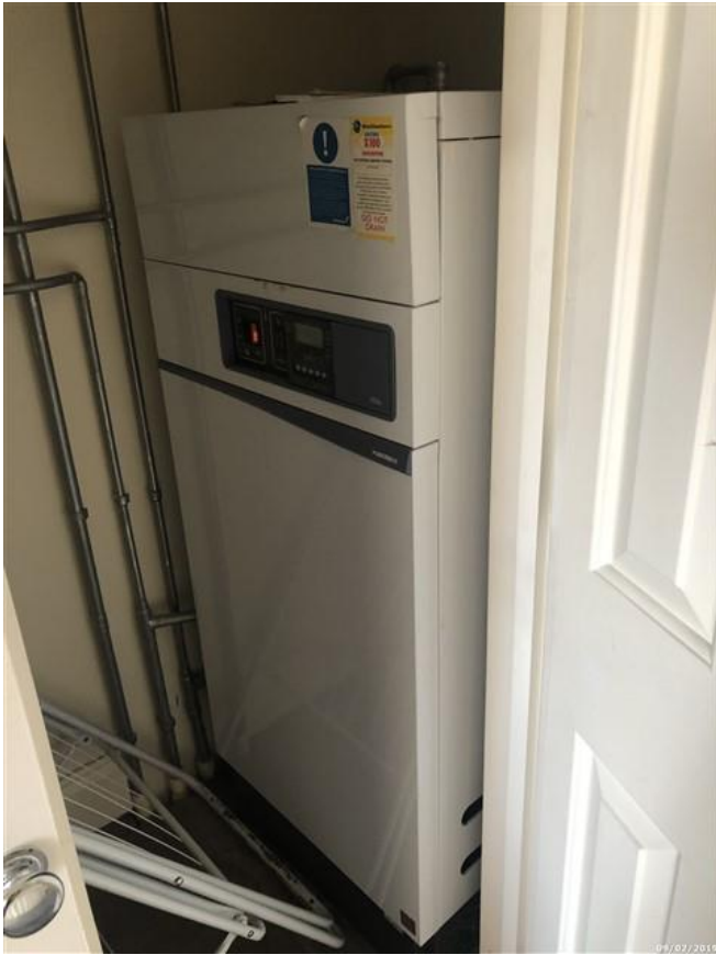
Images 8 & 9. A boiler with a thermal store: essentially a combination boiler, located in the airing cupboard off the second (top) floor landing. Make and model, along with model 'qualifier' (the specific model type) are clearly identifiable on the front panel of the boiler below.
