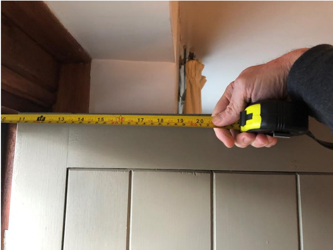
Image 5. Wall thickness of the main sandstone dwelling wall, measuring 480mm total.
