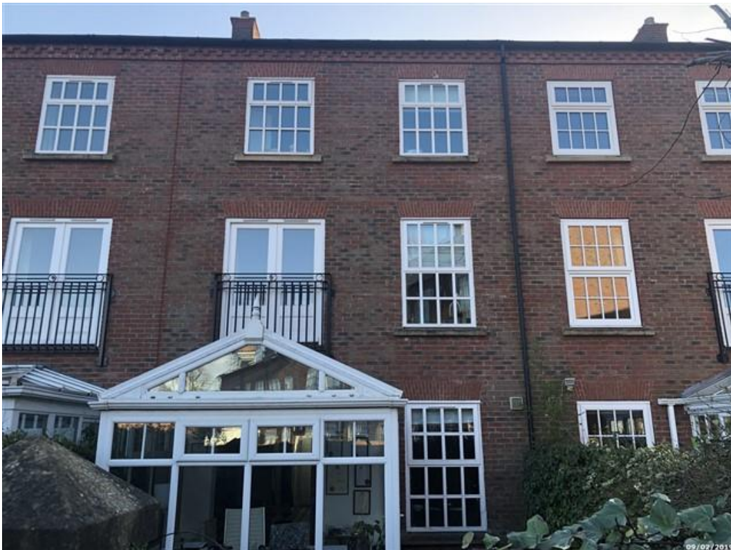
Image 2. Rear elevation of control property for phase 2 of the EPC study, showing conservatory, which is open to the main dwelling, and therefore considered a part of the dwelling
