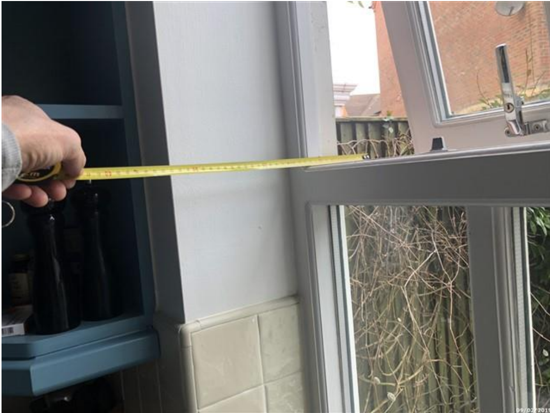
Image 5. Wall thickness of the timber framed wall, which throughout the property measures 310mm.
