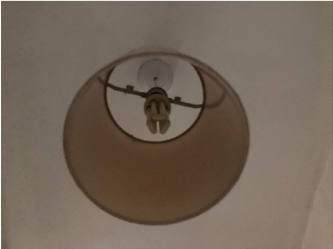
Image 13. Finally, a breakdown of fixed light fittings and low energy bulbs is requested within RdSAP.
