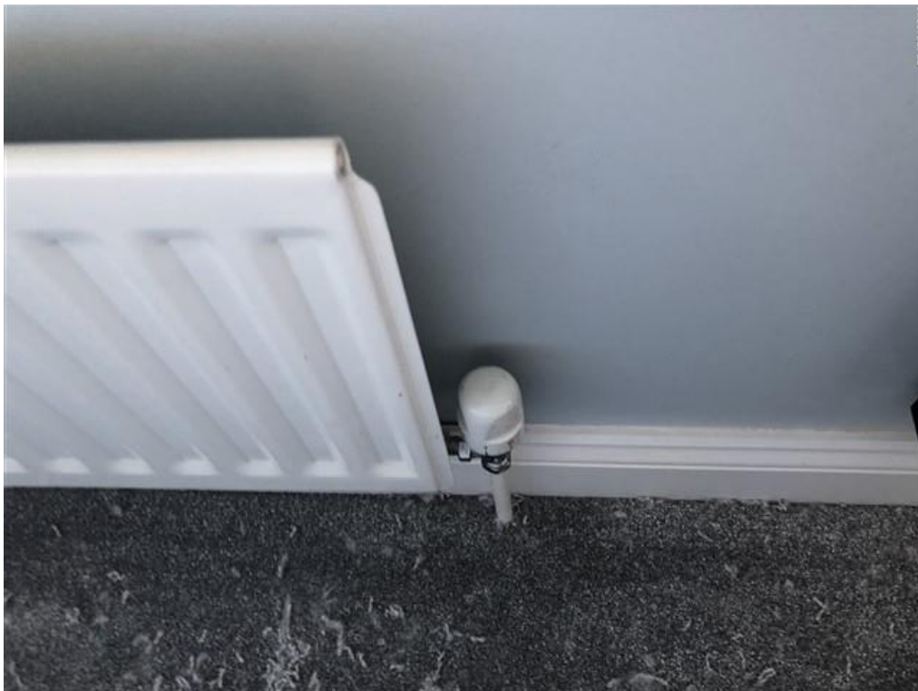
Image 11. Thermostatic radiator valves, or 'TRVs' are common. These allow the temperature of individual rooms to be adjusted, while the room thermostat will control the overall temperature of the dwelling from its central location.
