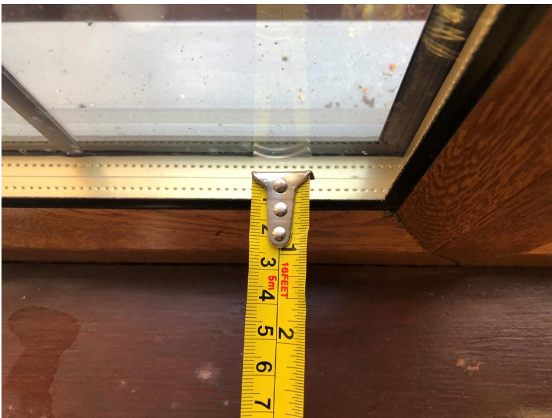
Image 12. The glazing gap is requested within RdSAP, as this can denote the efficiency, and possibly also the age of the glazing.
