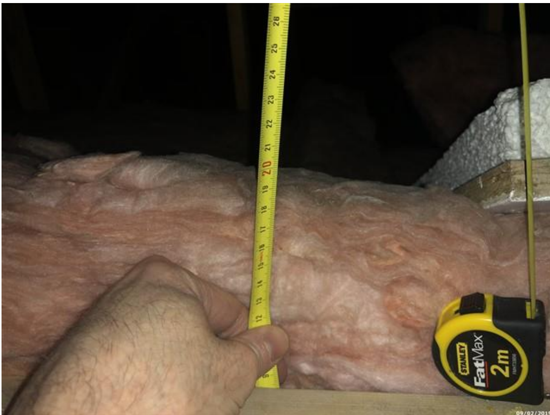
Image 6. Loft insulation, measuring 200mm
