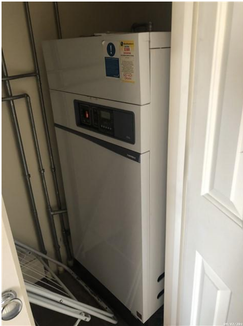
Images 4 & 5. A boiler with a thermal store: essentially a combination boiler, located in the airing cupboard off the second (top) floor landing. Make and model, along with model ‘qualifier’ (the specific model type) are clearly identifiable on the front panel of the boiler below.
