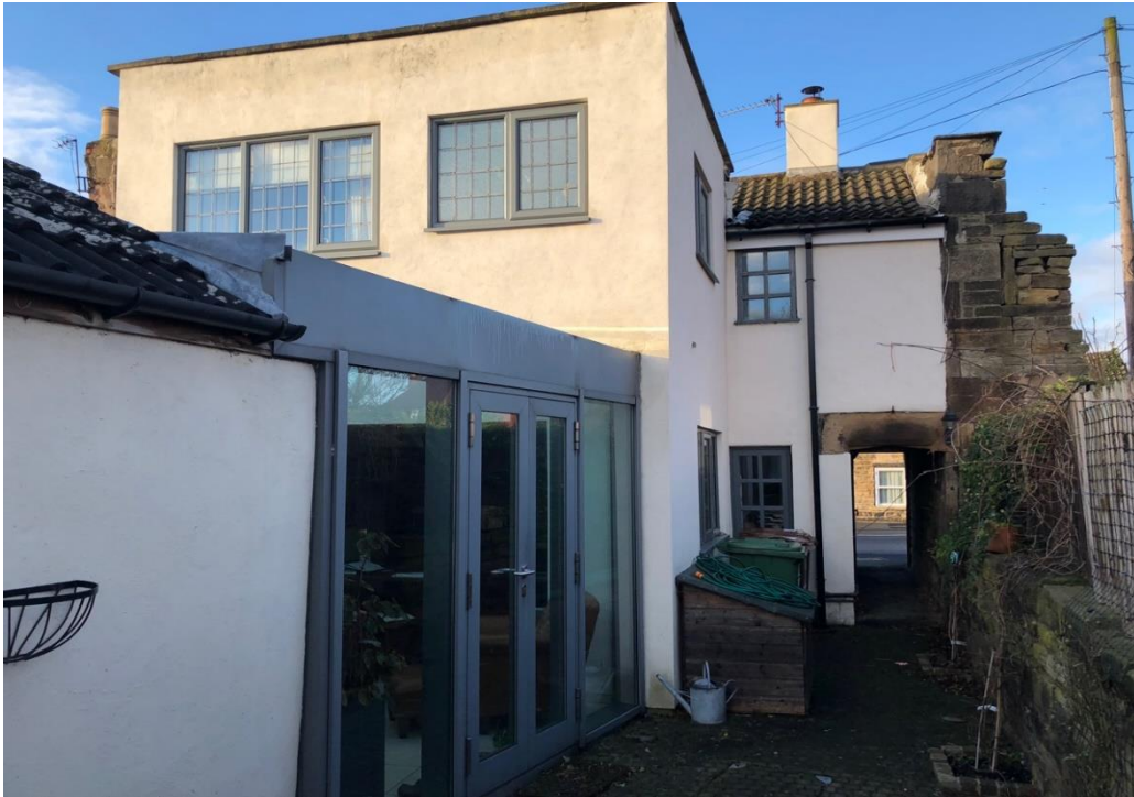
Image 2. Rear elevation of control property for phase 1 of the EPC study, showing two storey circa 1970 extension, and glazed kitchen extension beyond this. The building that adjoins the kitchen extension to the left hand side of this photograph belongs to the neighbouring property.
