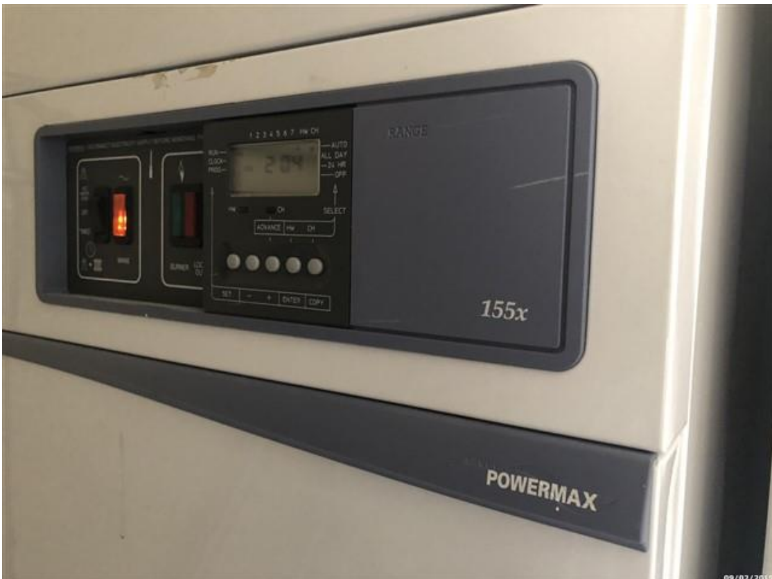
Images 8 & 9. A boiler with a thermal store: essentially a combination boiler, located in the airing cupboard off the second (top) floor landing. Make and model, along with model 'qualifier' (the specific model type) are clearly identifiable on the front panel of the boiler below.
