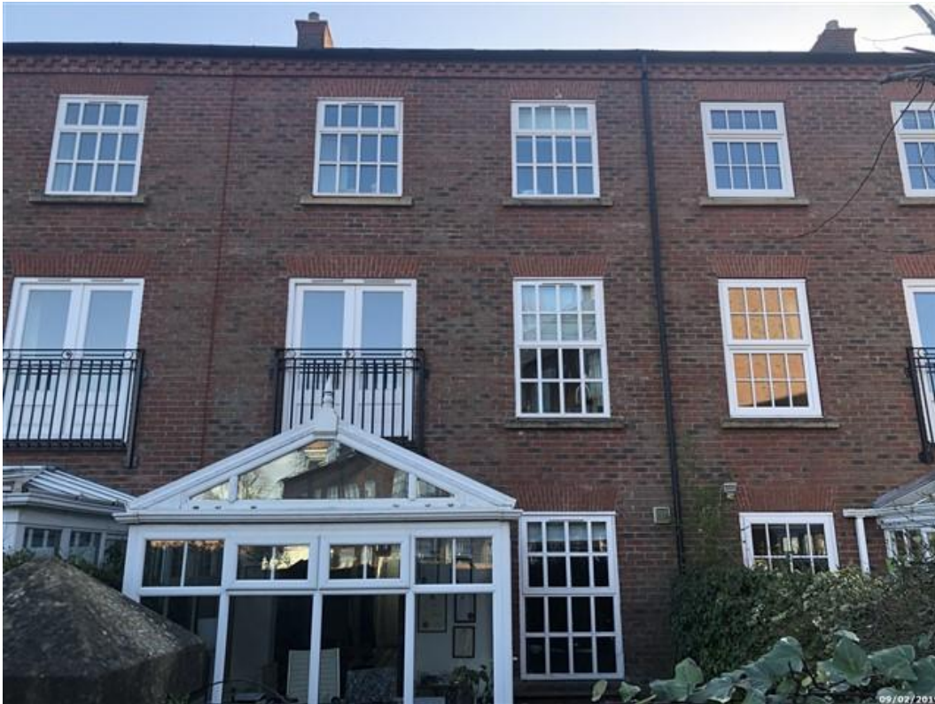
Image 2. Rear elevation of control property for phase 2 of the EPC study, showing conservatory, which is open to the main dwelling, and therefore considered a part of the dwelling
