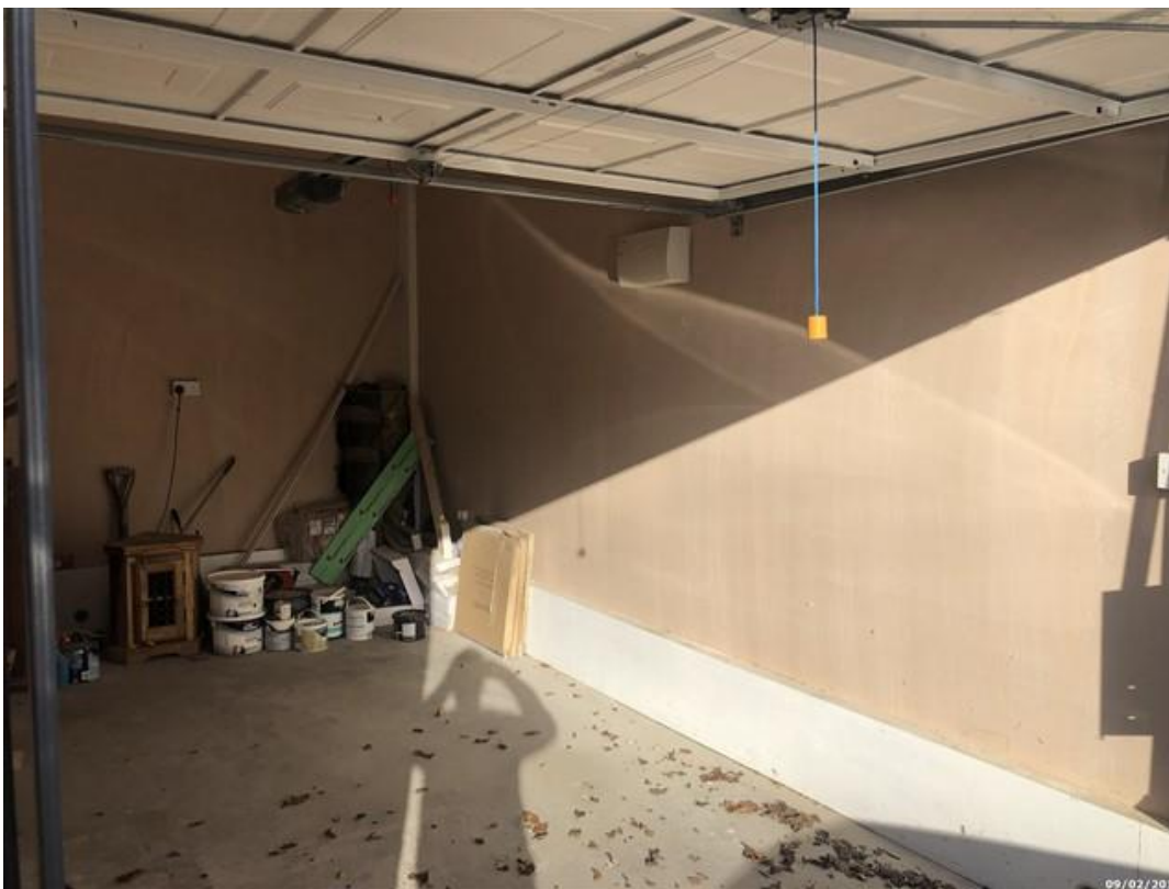
Image 4. Internal perimeter of the integral garage: this is considered an exposed, external wall according to RdSAP conventions.
