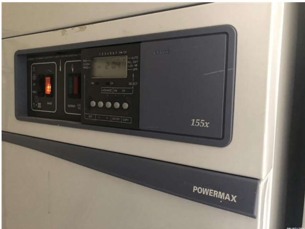
Images 4 & 5. A boiler with a thermal store: essentially a combination boiler, located in the airing cupboard off the second (top) floor landing. Make and model, along with model ‘qualifier’ (the specific model type) are clearly identifiable on the front panel of the boiler below.
