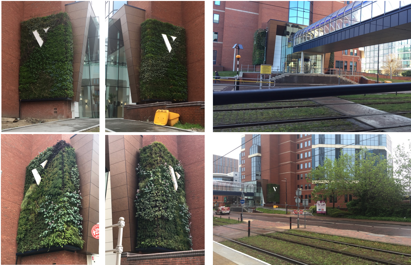
Figure 3. Victoria. A living wall placed on both sides of the Victoria Building, Media City, Salford. It is a recent development (2019) with the plants not in leaf at the start of the observations (October 2019) (top left) and in leaf after (July 2020) (bottom left). The wall is presented with a 'V' for the company's name, and placed slightly above ground, mirroring the entrance (top right). It was adjacent to a main road and tramway and street trees placed side of the building (bottom right).
