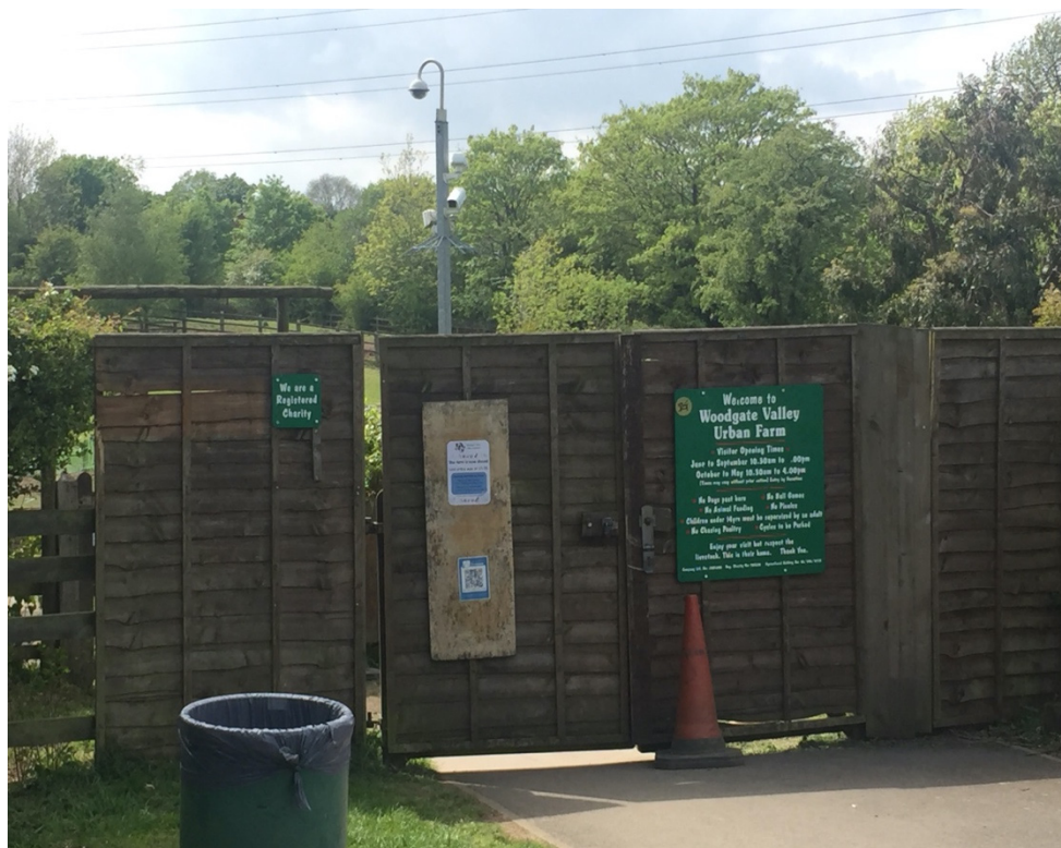
Figure 2. CCTV systems installed at an urban farm experiencing vandalism.
