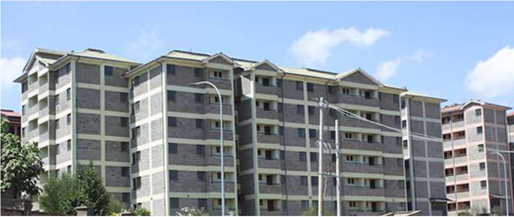
Figure 3 Kibera 3000 housing upgrading project (Source: Correspondent, 2016)
