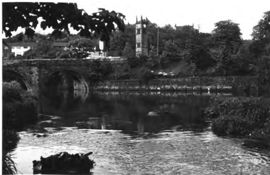
Plate 8. Site 8, Ringly, viewed from downstream.
