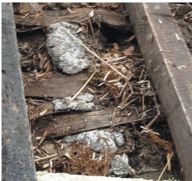
Figure 11. Laths bonded to plaster uncovered during re-thatching in July 2019. Image copyright Anthony Simpson.
