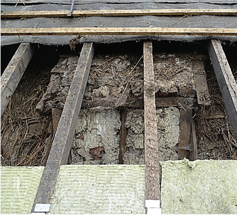
Figure 10. Infilled dormer-type window frame uncovered during re-thatching in July 2019. Image copyright Anthony Simpson.
