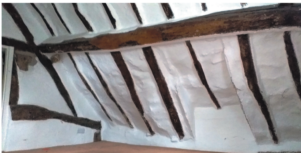
Figure 6. Internal view of south facing roof timbers and daub surface. Image copyright South Trafford Archaeological Group.
