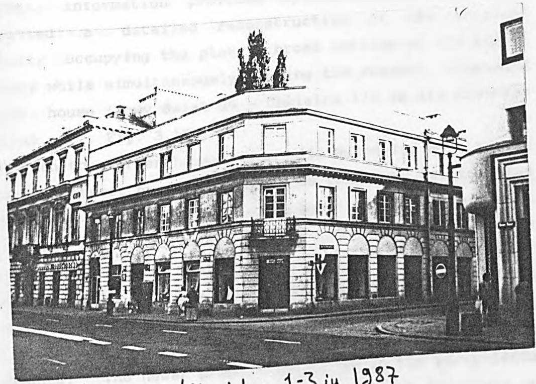
Figure 3.15 Readaption and post-war vertical extension of I. Gajewski's town-house
