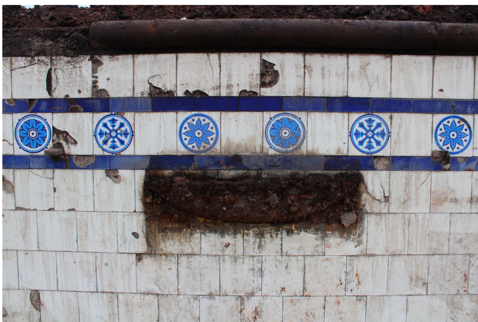
Figure 10. Examples of the two-tone motif tiles used in the first-class pool at Mayfield Baths, together with one of the cast-iron spittoons (© University of Salford).
