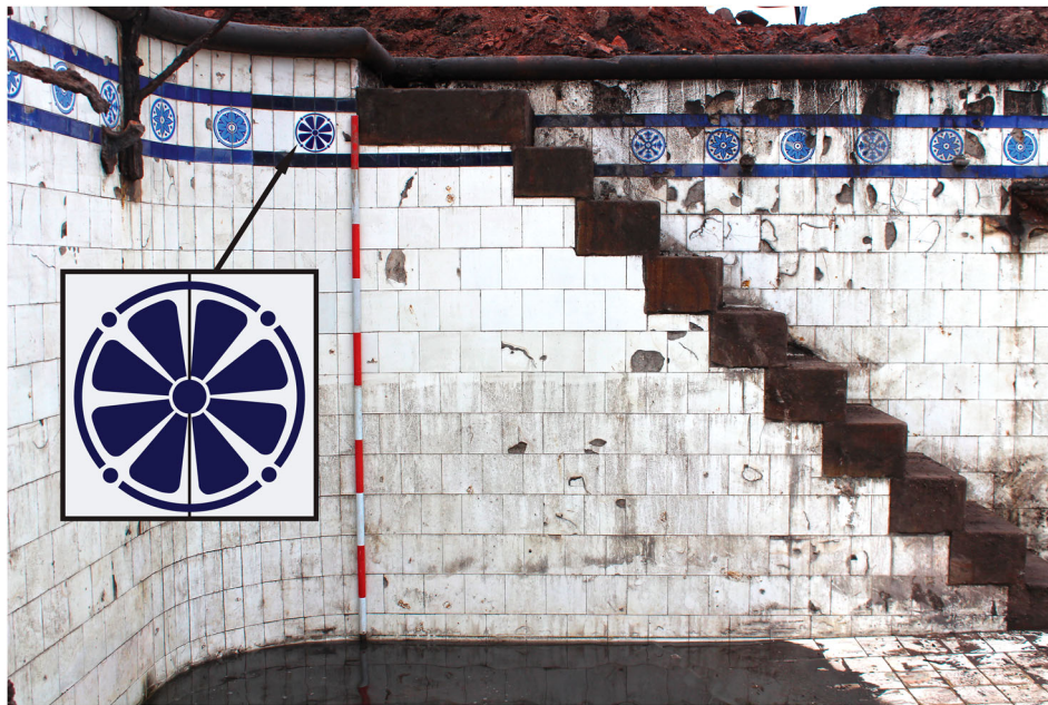
Figure 11. The inserted steps in the first-class pool, with later monochrome radial tile (© University of Salford).
