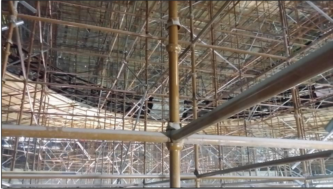
Figure 15: Large scale scaffolding on the transport project 36
