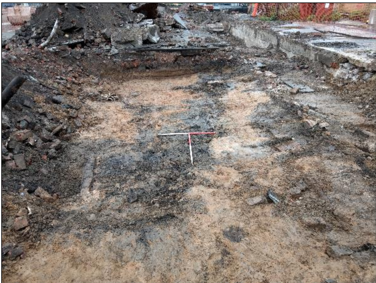
Plate 9: Extension to Trench 3 showing the foundation trench for drain 303
