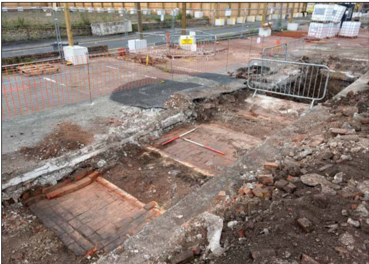
Plate 5: Boiler remains associated with the 20 th -century rubber works
