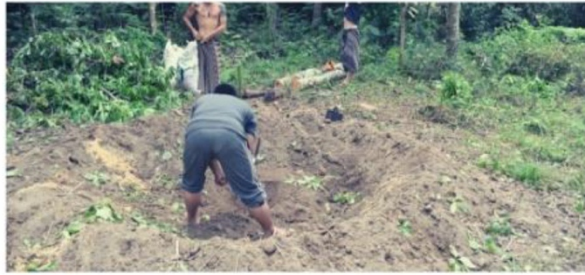
1 A pit 1 m in depth is prepared
