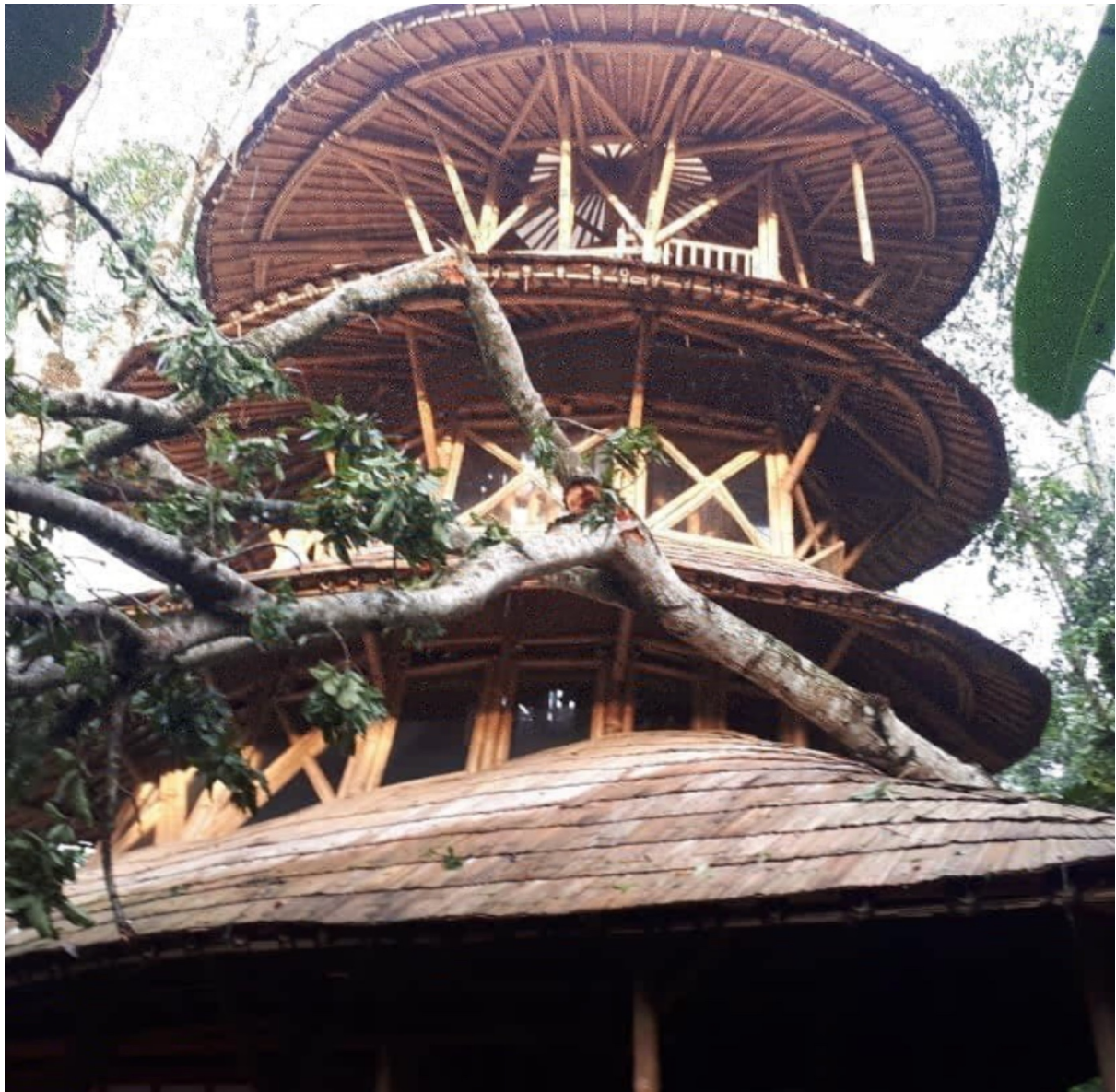
Box 7: Evidence of the incident displaying the bamboo towers structural integrity after a storm, Source, Yayasan Bringin Foundation (Omah Lor owner)
