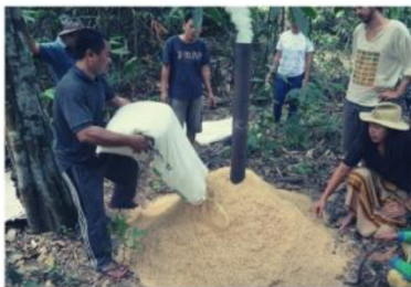
3 Dried rice husk added to smother the fire within the reactor
