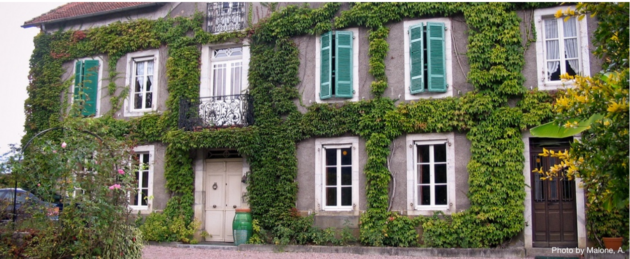
Vines on trellises provide a quick and easy way to reduce wall temperature
