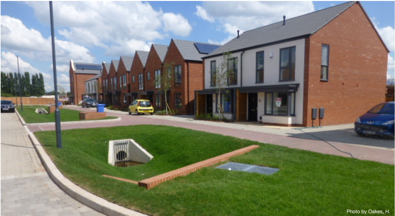
Swales in Manor Kingsway Phase 1, Derby work to reduce flood risk
