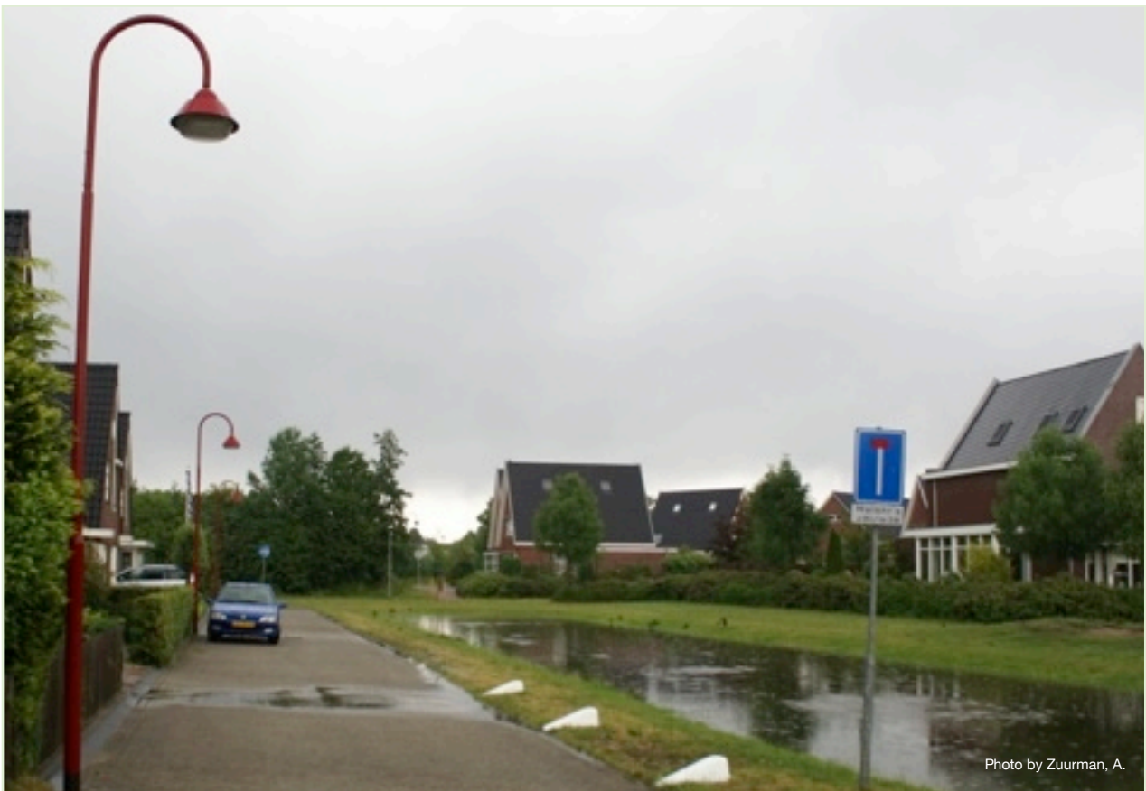
Designing infiltration basins into developments can greatly reduce property damage during flood events
