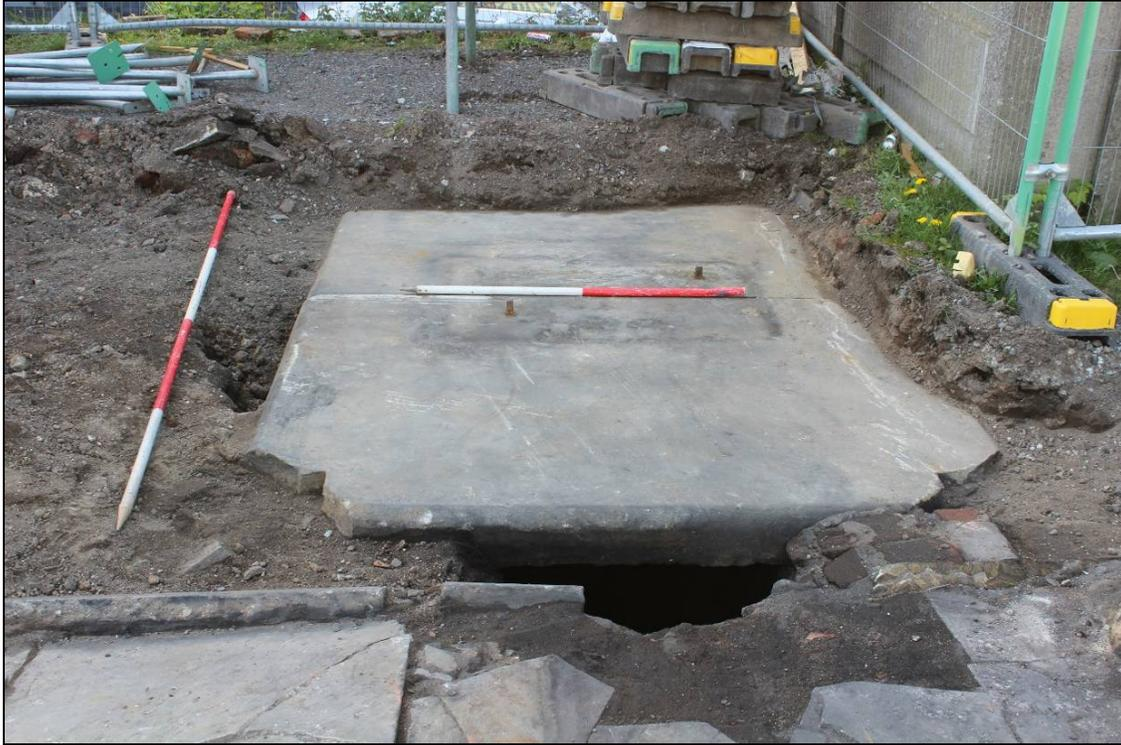
*Plate 40: Stone slabs sealing William Cowherd's vault*
