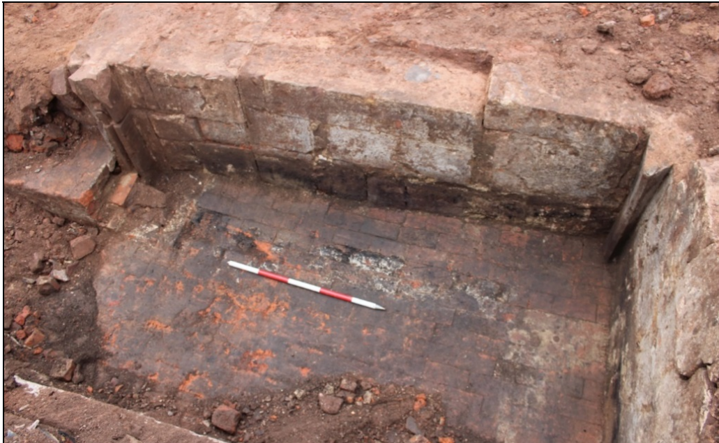
Plate 54: Rib-vaulted cellar looking south (1m scale)
