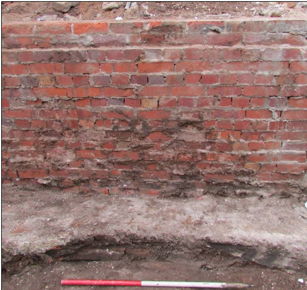
Plate 15: South-facing elevation of modern brick wall 306 (0.5m scale)
