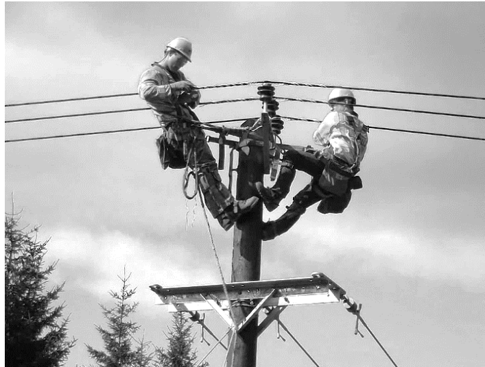
Figure 1.2: Overhead line workers fixing an overground cable fault (Source: SSE [93])
