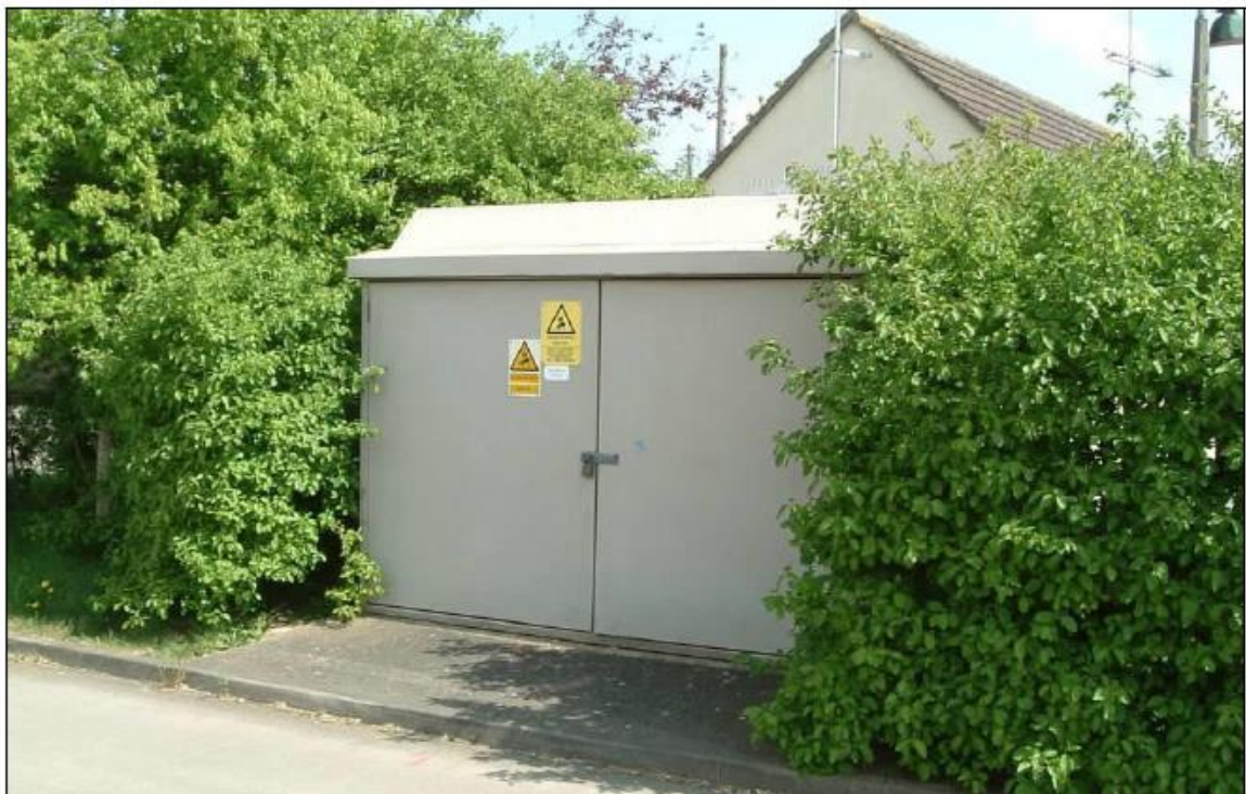
Figure 2.5: Distribution substation with equipment operating at 11kV and 400/230 volts (Source: SSE [7])
