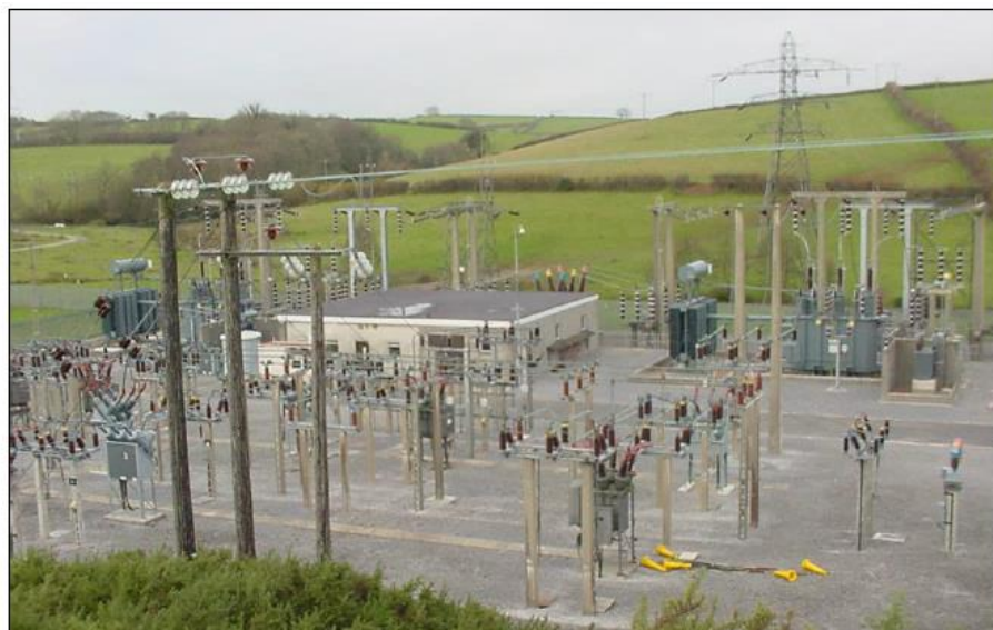
Figure 2.3: 132kV Grid Substation showing 132kV terminal tower and the start of 33kV wood pole overhead line (Source: SSE [7])
