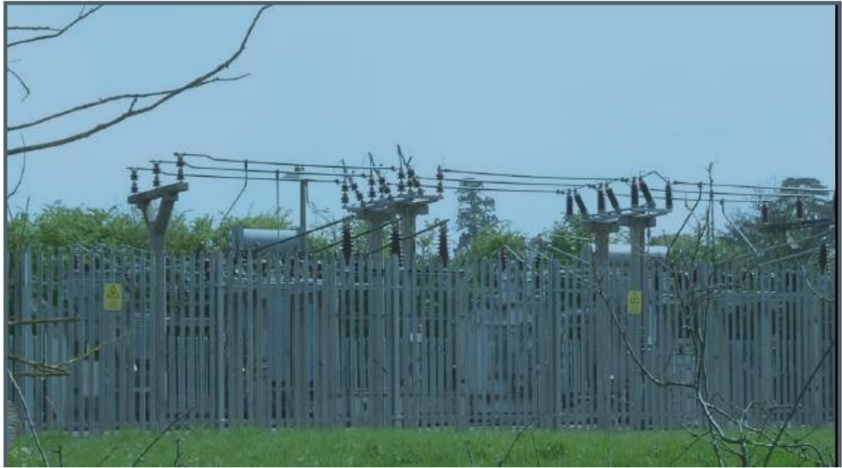
Figure 2.4: Primary substation showing equipment operating at 33kV and 11kV (Source: SSE [7])
