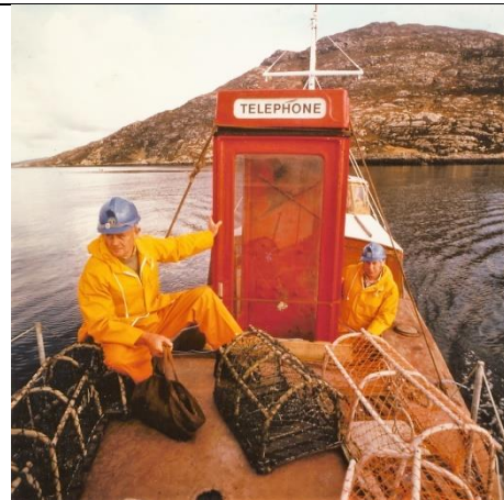
Fig 12. This picture taken in 1983 shows a new pre-assembled K8 kiosk being delivered to a remote Scottish isle, to serve 200 people. (Photograph courtesy of BT Heritage & Archives. BT image TCB 417/E77001)
