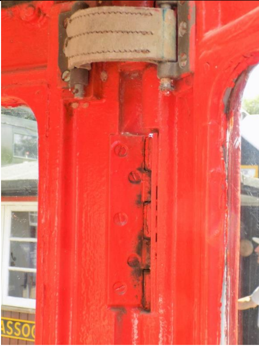
Fig 9. Brass hinges were used to support the K8 door rather than pivot bolts as favoured by Bruce Martin. The leather strap limits the extent to which the door can be opened. Picture taken 2018.
