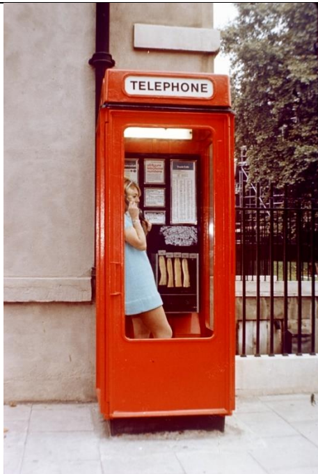
Fig 11. This picture taken in 1970 of a woman using a K8 kiosk clearly shows the always-on fluorescent tube light. (Photograph courtesy of BT Heritage & Archives. BT image TCB 473/P10607)
