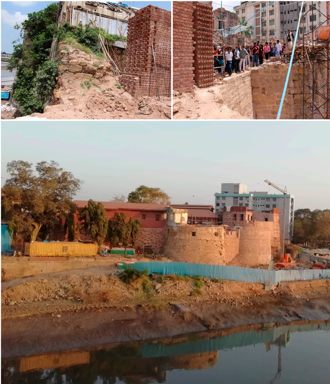
Figure 7. Redevelopment occurring alongside the old Surat fort walls.
