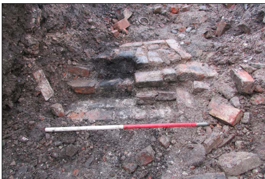
Figure 21. Walls (008) and (009), in the foreground and background respectively, showing black staining. Looking east.
