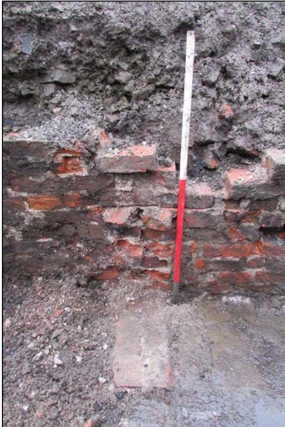
Figure 31. Remains of the southernmost brick buttress in wall (077). Looking north.
