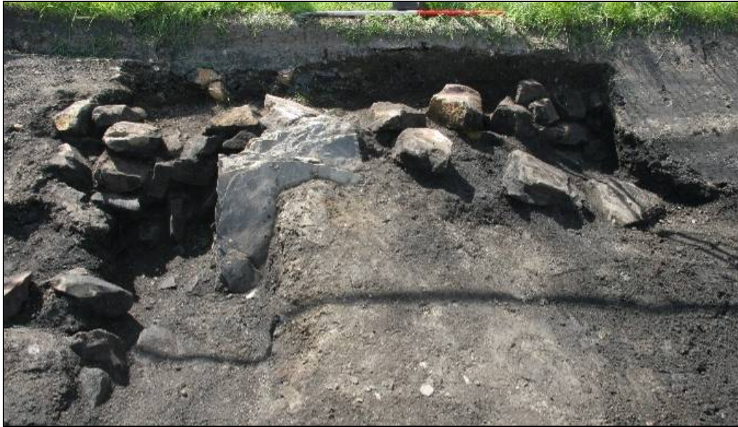
Plate 44: Section of stone feature, which was associated with the construction and drainage of the current public footpath
