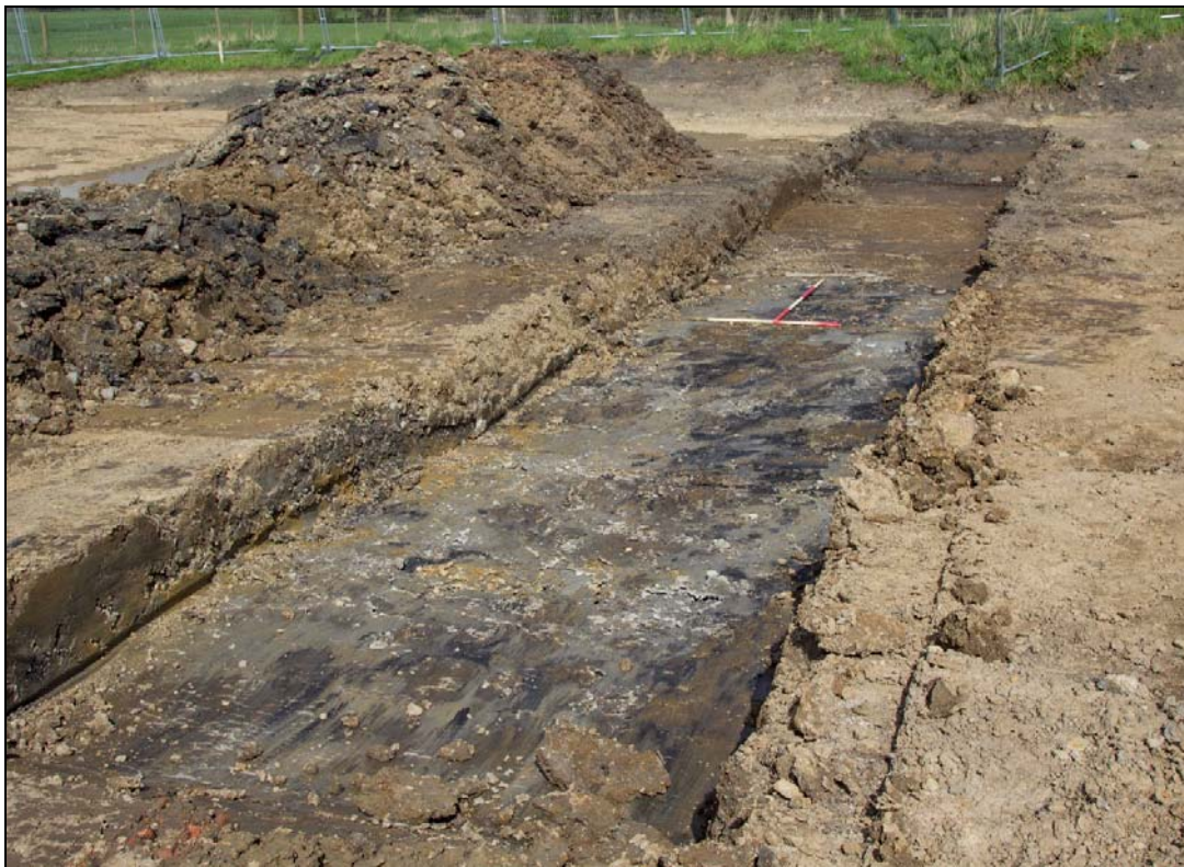
Plate 32: Machine-excavated sondage to the north of Area B1, looking east
