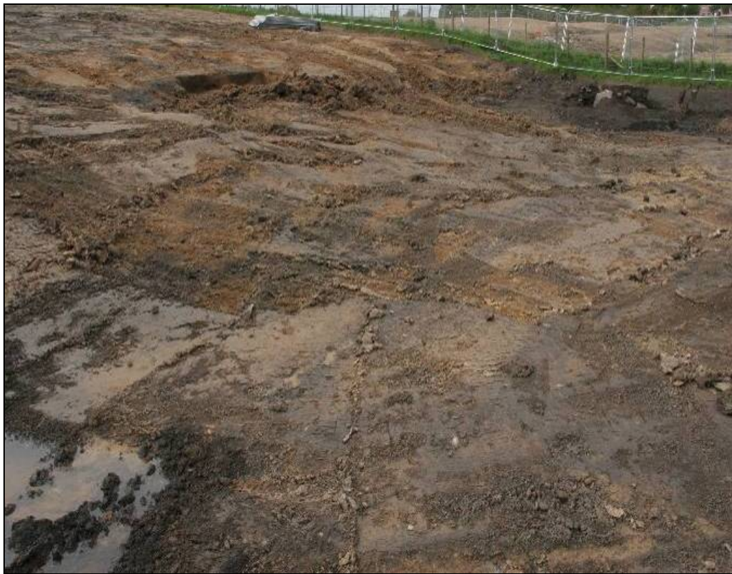
Plate 45: General view of Area C, looking south-west
