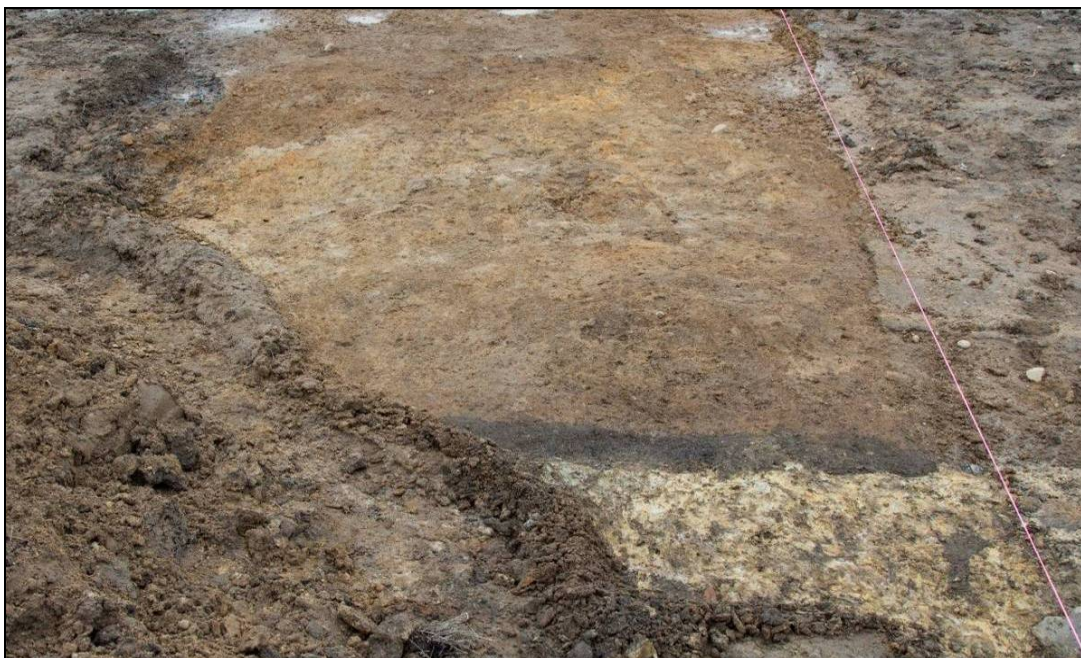
Plate 8: Pre-excavation view of ditch [108] and re-cut [110], looking west
