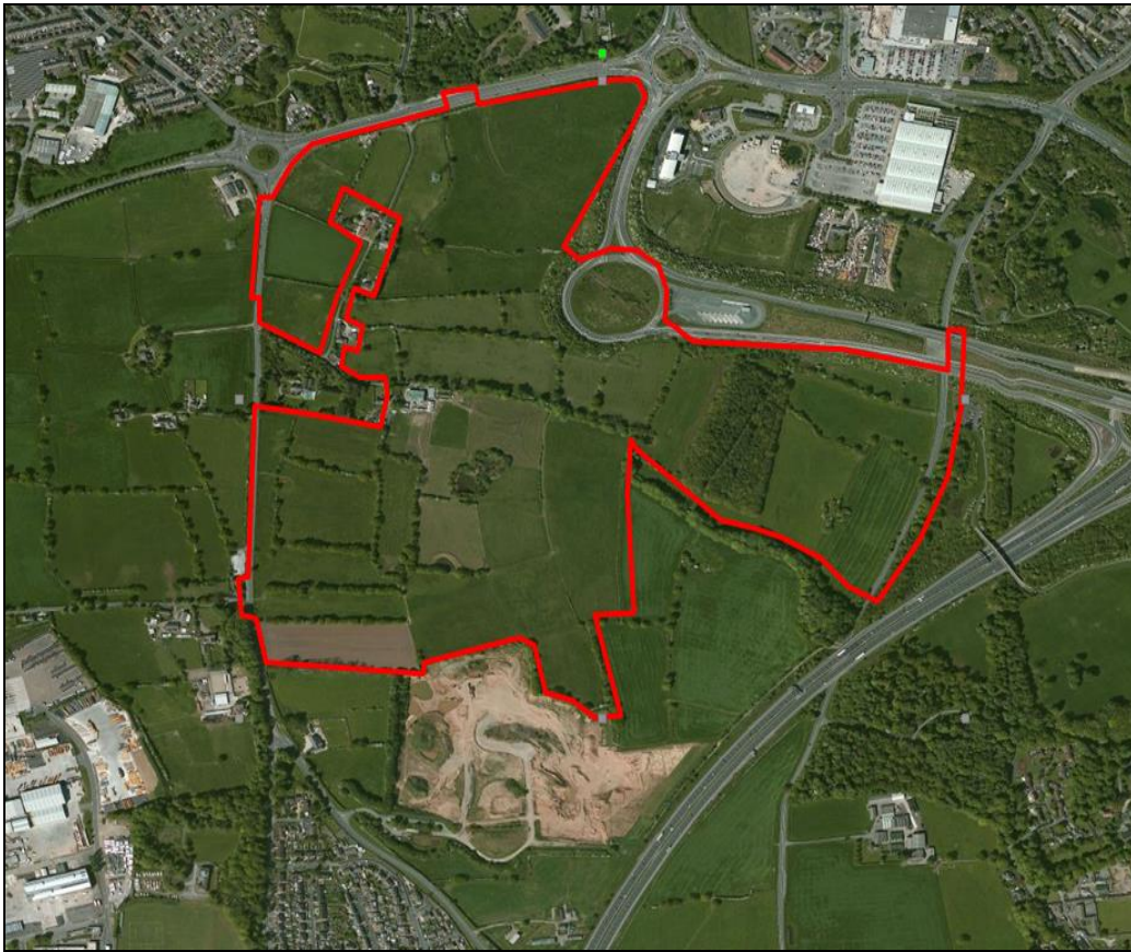
Plate 1: Aerial view across Cuerden, showing the site boundary
