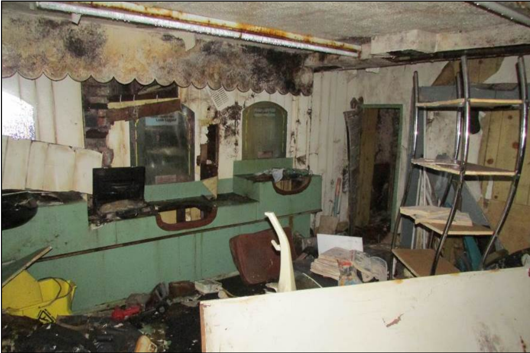
Plate 8: The interior of the basement, showing the modern alterations
