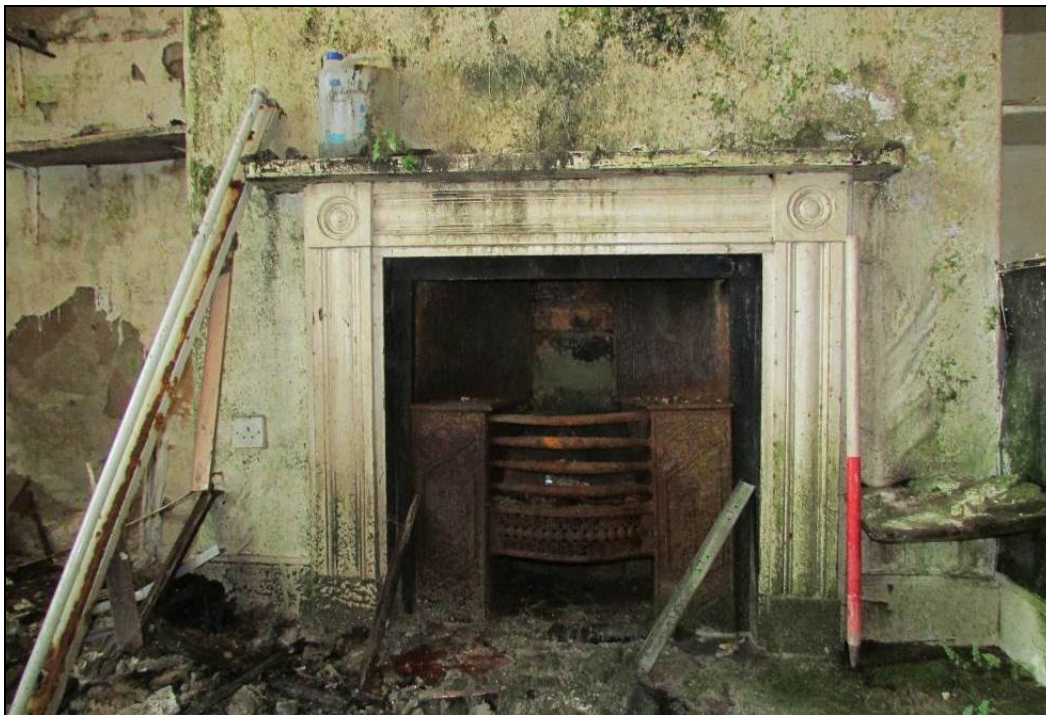
Plate 11: Fireplace detail in the second room on the first floor
