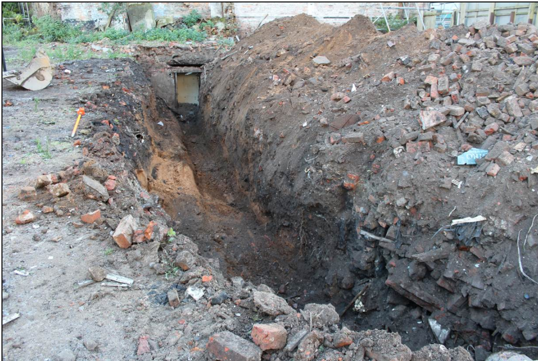
Plate 14: General view of the excavated trench, looking south-east
