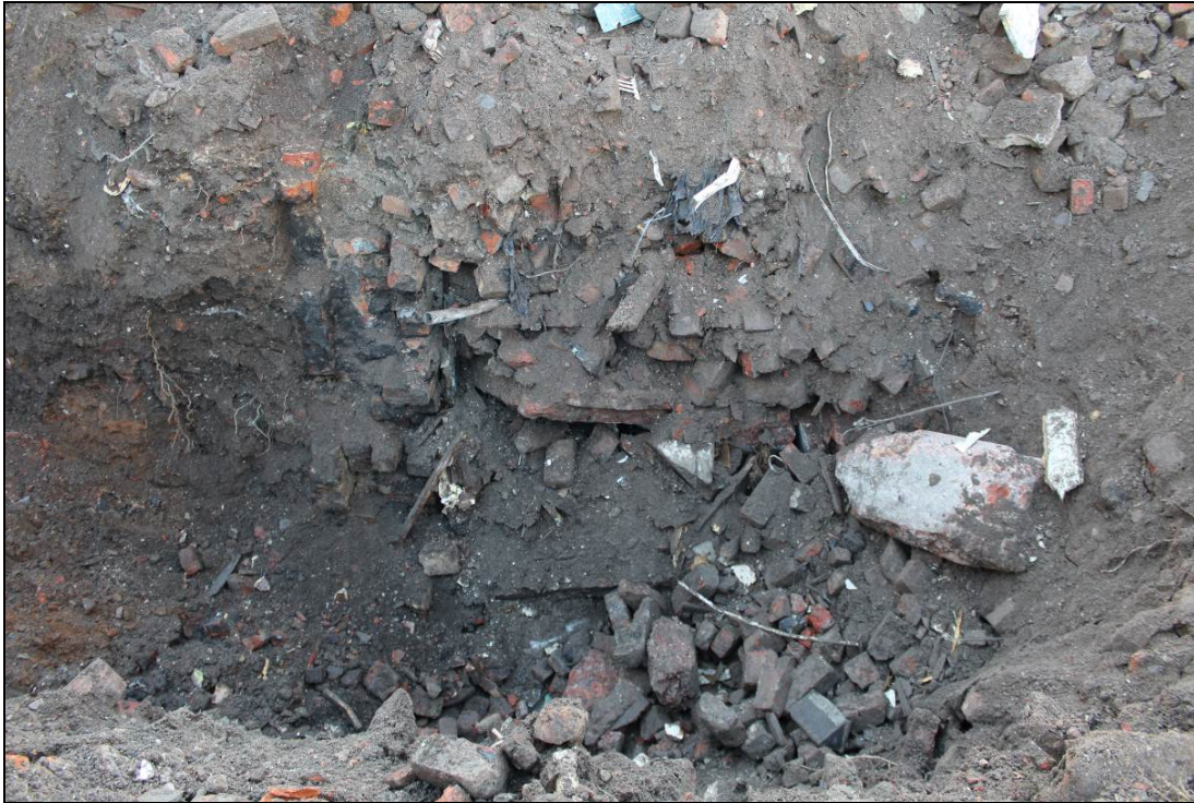
Plate 16: Rubble filled north basement, looking west
