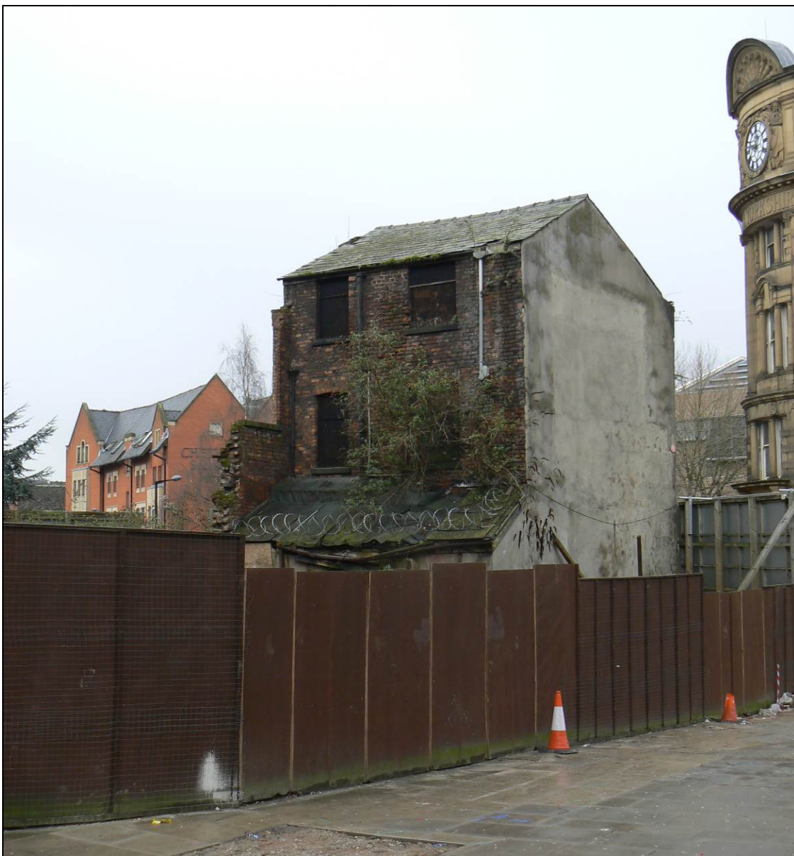
Plate 3: North-east and south-eastern elevations, looking north-west
