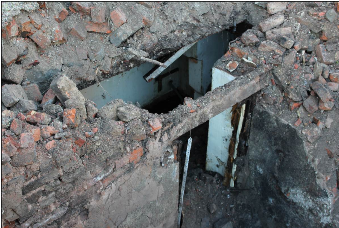
Plate 15: South-east basement, looking south
