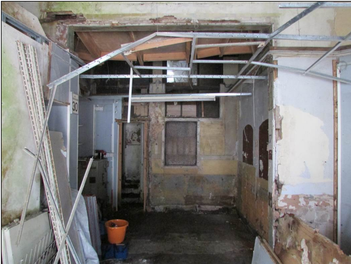
Plate 5: The interior of the main room on the ground floor
