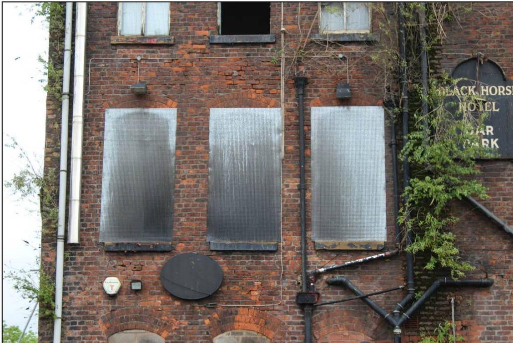
*Plate 17: The blocked-up window apertures on the first floor*
