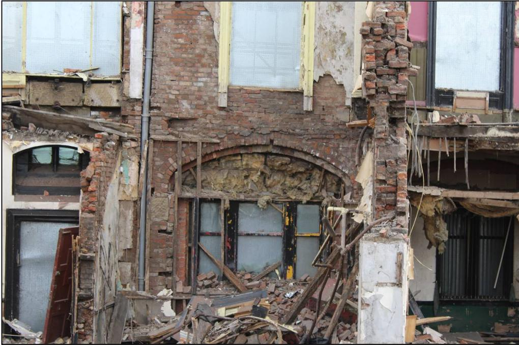
*Plate 22: The internal view of the blocked-up archway in the northern elevation*
