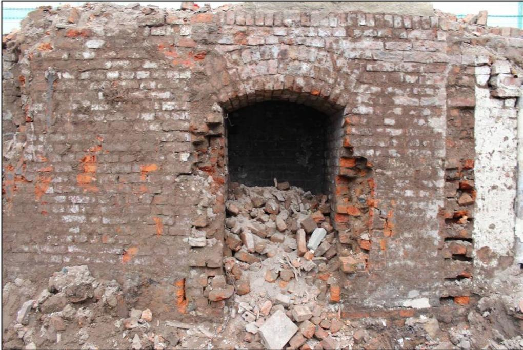
*Plate 24: The blocked-up doorway within the cellar's northern wall*
