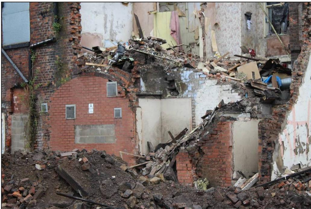
*Plate B17: Detail of the blocked-up archway in the southern façade*
