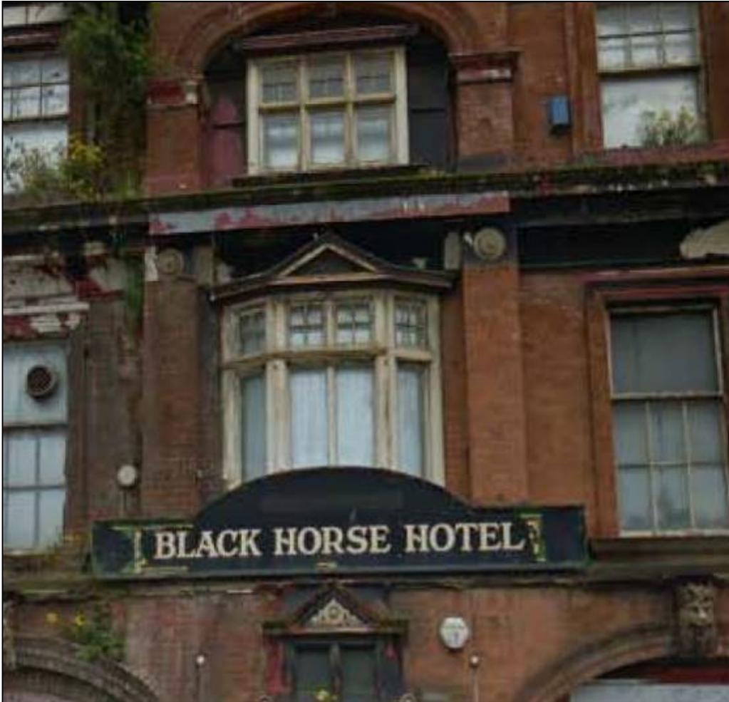
*Plate 9: The canted oriel window on the first floor*
