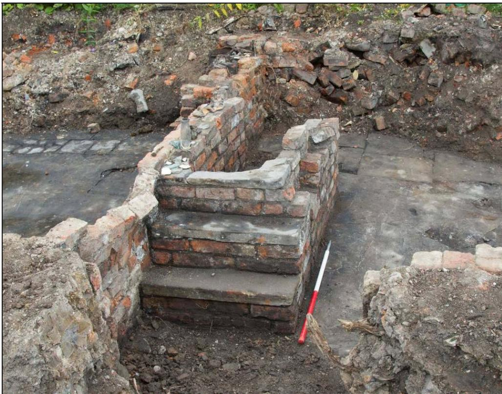
*Plate 110: House 11 staircase 4009 built against wall 4008, looking east*
