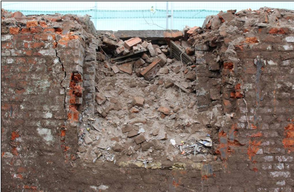
*Plate 23: Blocked cellar light within the northern elevation*
