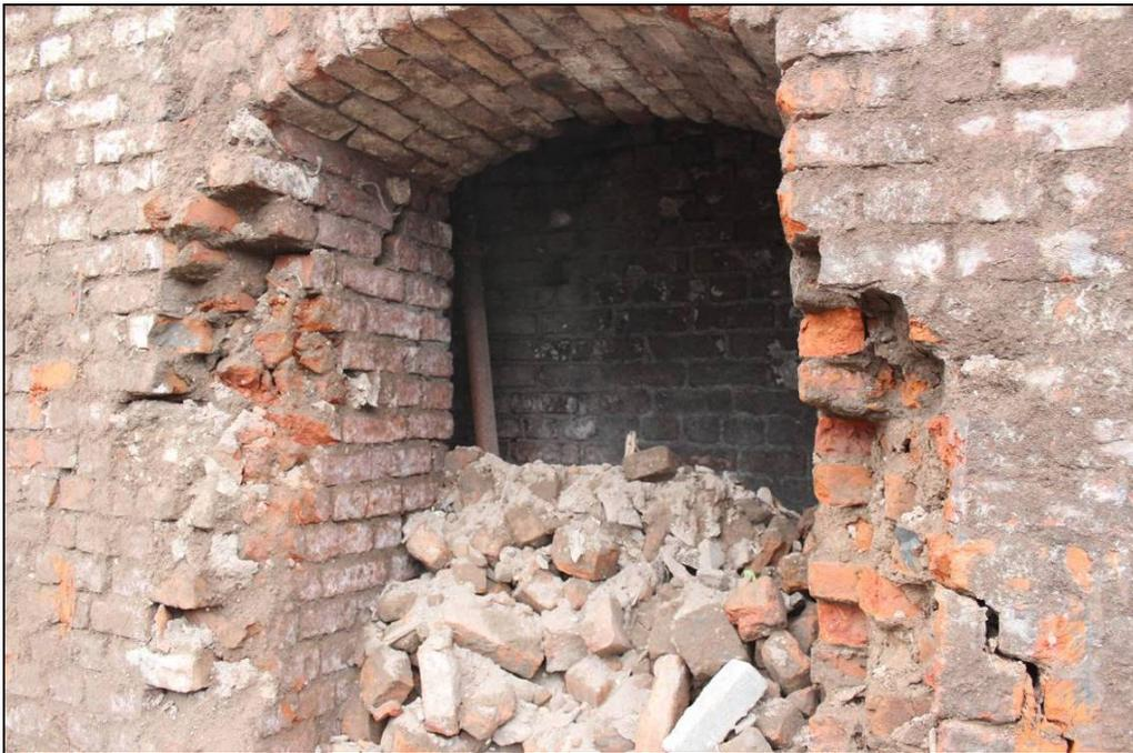
*Plate 25: Detail of the blocked door and passageway leading up to street level within the northern wall*
