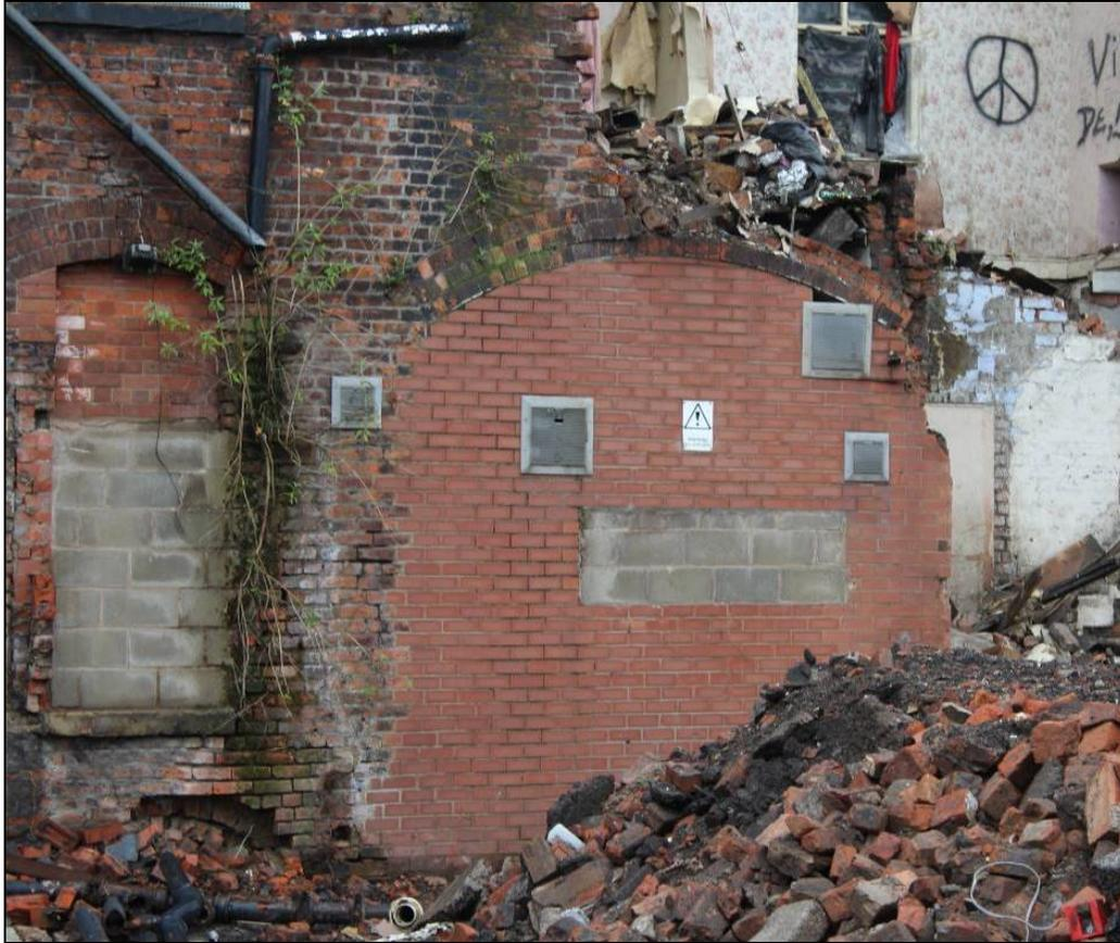
*Plate 16: The blocked-up archway at the eastern end of the southern façade*
