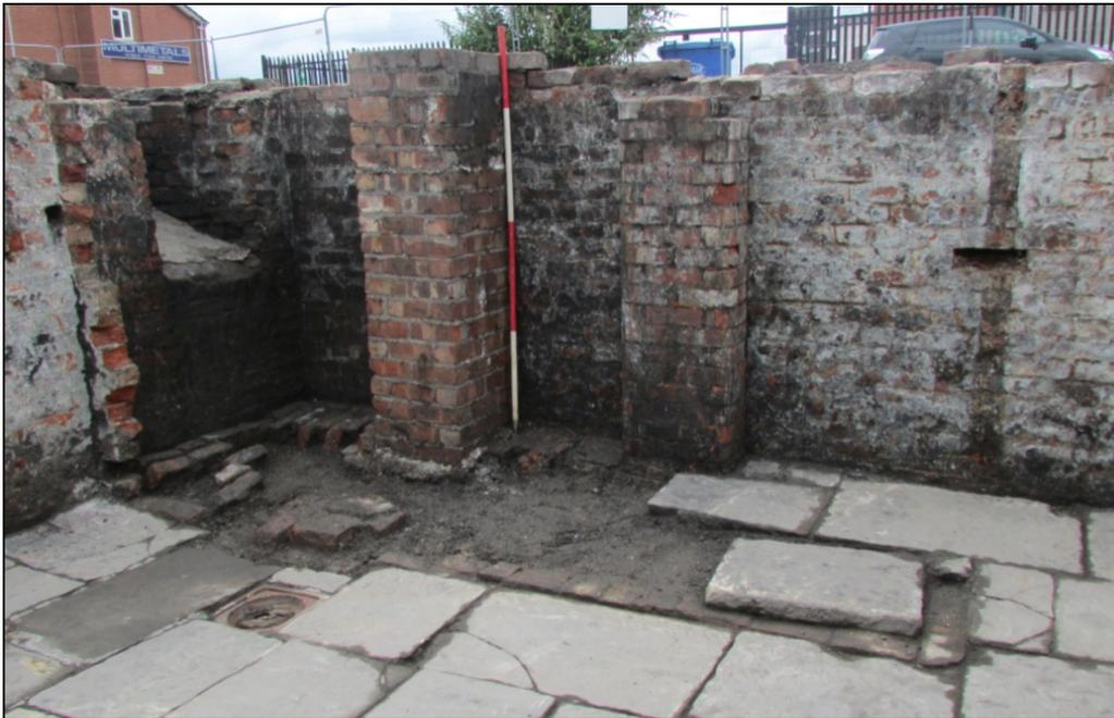
*Plate 61: The base of single-skin wall 2057 and buttresses 2054 and 2055*
