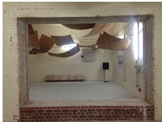
Figure 4.11: Large reverberant room ( 5s RT_{60} )
