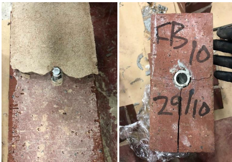
Fig. 5. Failure mechanisms identified in a) bar reinforced, and b) tube reinforced triplets [12].
