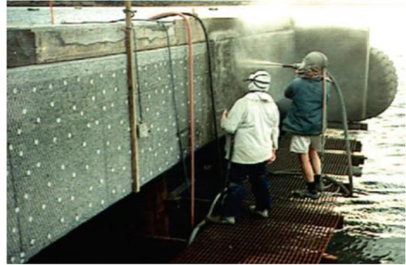
**Figure 2.15** Application of Ti/MMO anode and mortar cover (Araujo et al., 2013).
