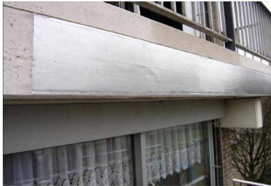
**Figure 2.12** Application of zinc sheet anode in SACP for RC structure
