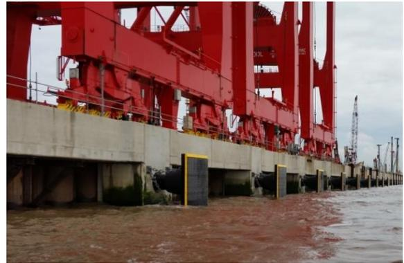
**Figure 2.16** Application of ICCP to protect the steel tubular piles.
