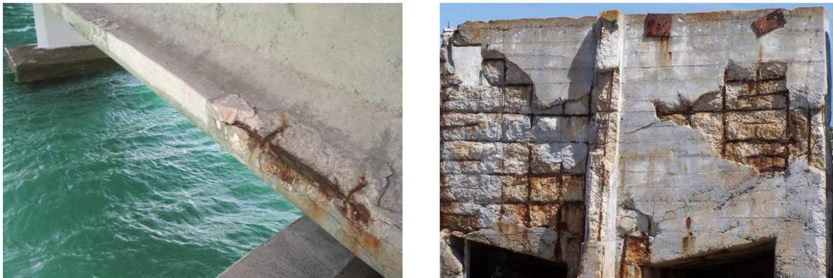
**Figure 2.1** Schematic illustration of steel corrosion in offshore RC structures.
