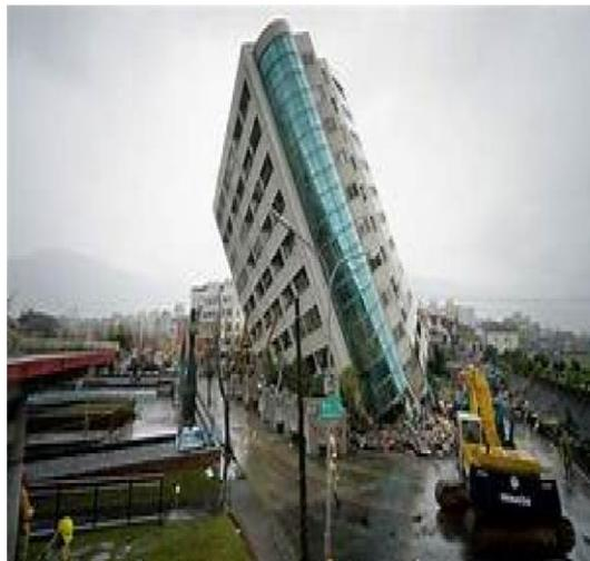
**Figure 2-1 Building tilted by ground failure caused by soil deformation (Taiwan earthquake, 2018)**
