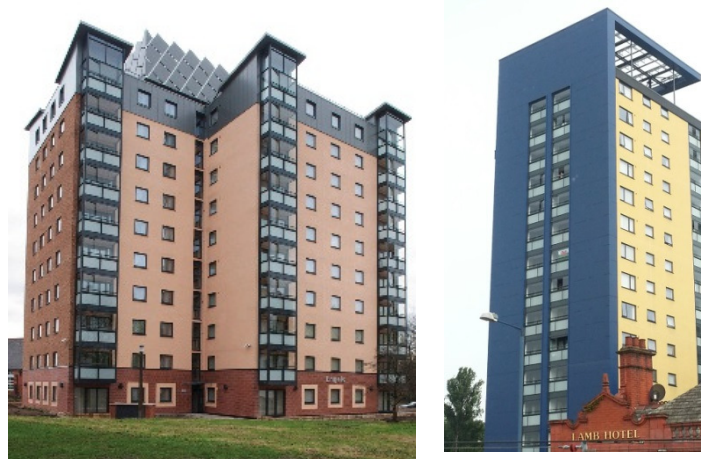
Figure 7.19: City West Housing Trust high rise blocks after works
