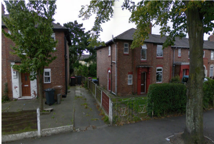
Figure 7.8: City West Housing Trust environmental-led programme before works
