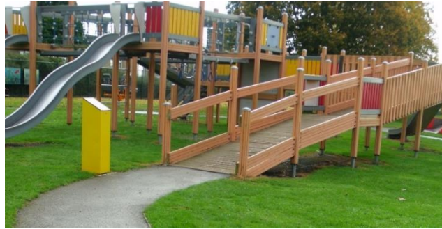
Figure 8.116 Ramped access to platform
