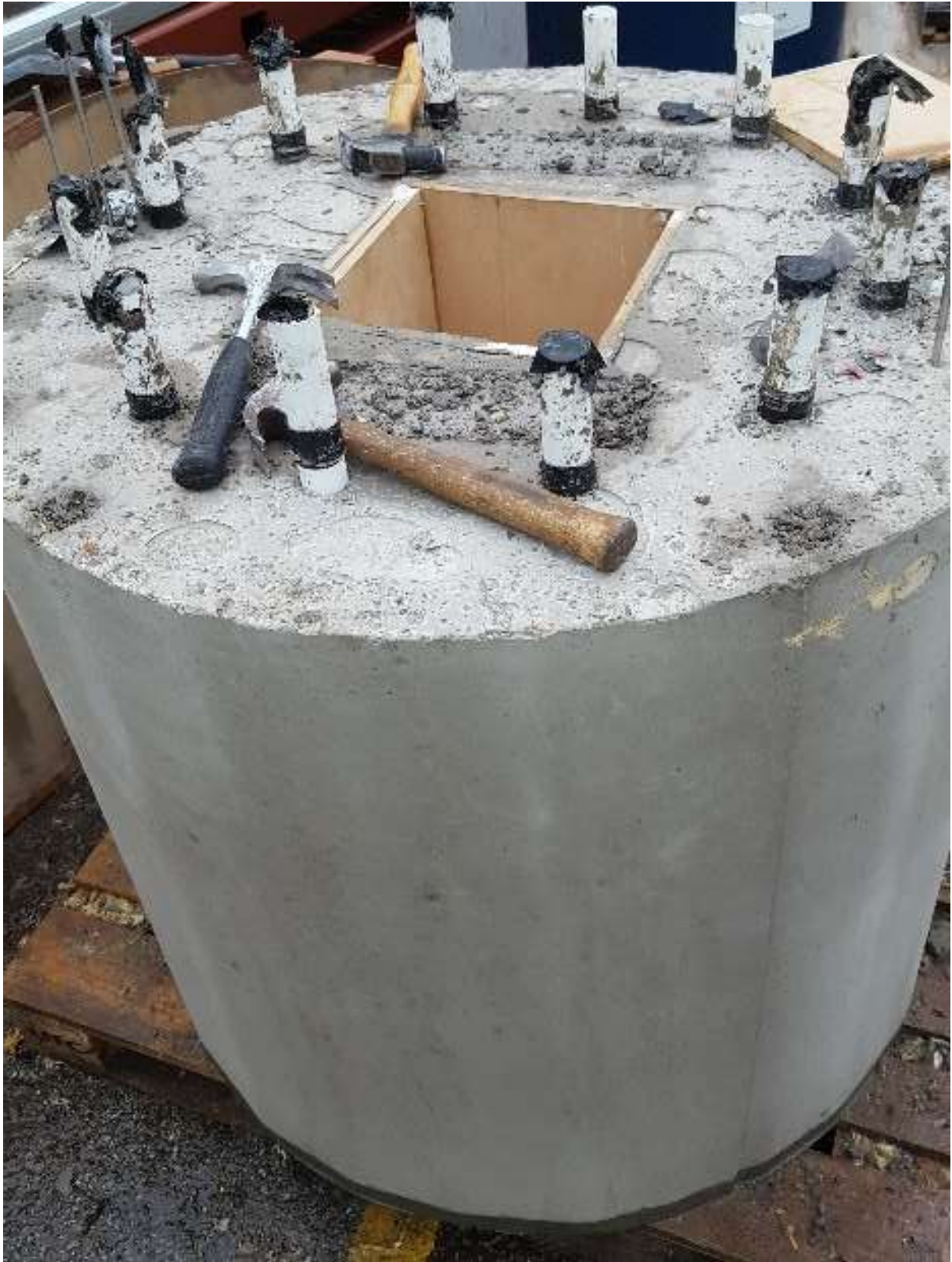
Figure 3-23: Concrete structure, as built, being removed from its foam.
