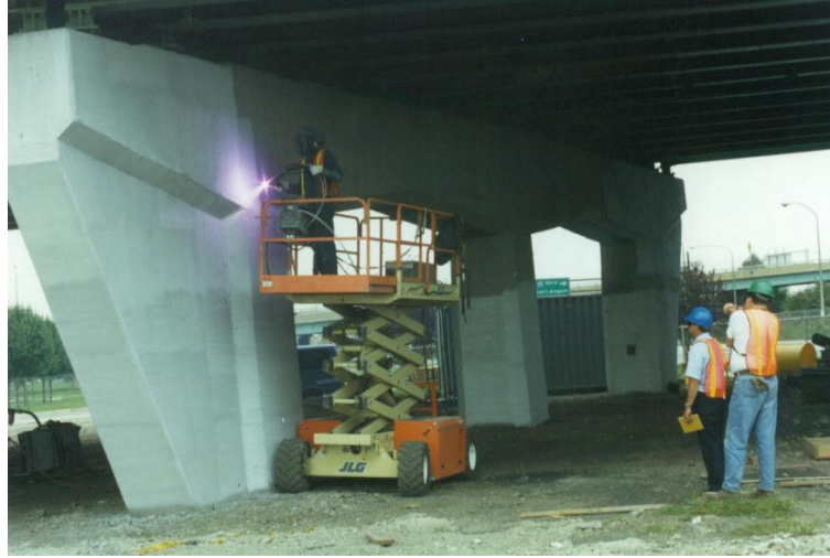
Figure 2.27: A sacrificial coating of Al-Zn-In to a reinforced concrete bridge pier, (Daily, 1999).
