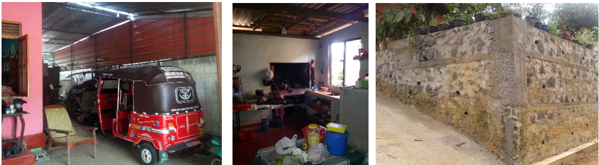
Figure 3: Examples of modifications carried out by occupants in post-tsunami houses
