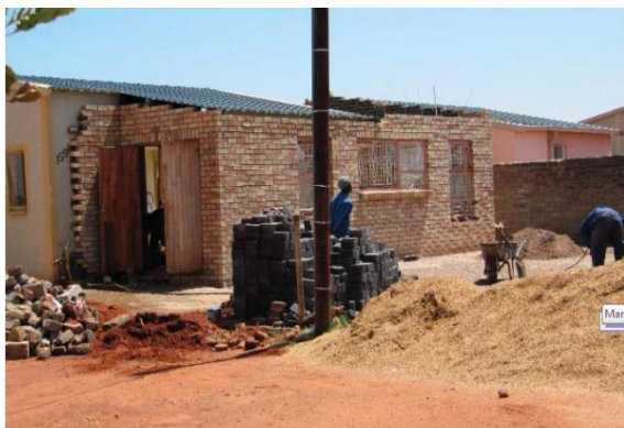
Figure 3-4: Incremental building in Progress
