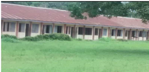
Figure 1: Open Ventilation System used
