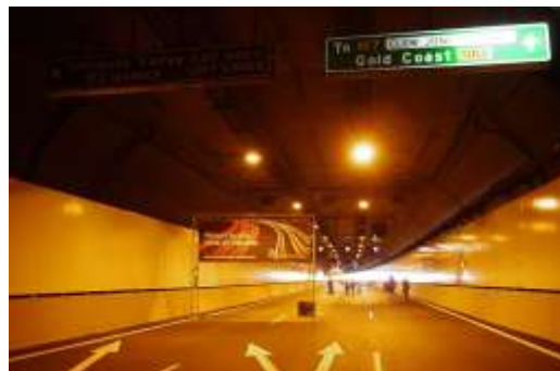
Road tunnel Brisbane Australia (6).
