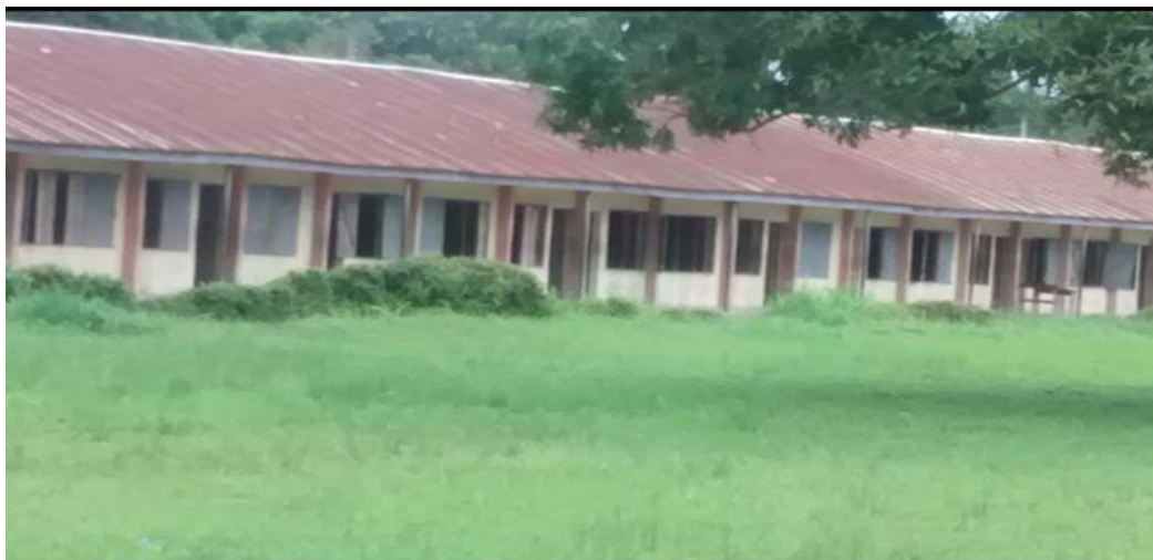
Figure 2.14 Open windows and Door as Ventilation System used in Public Schools Source: Field Work (2015)
