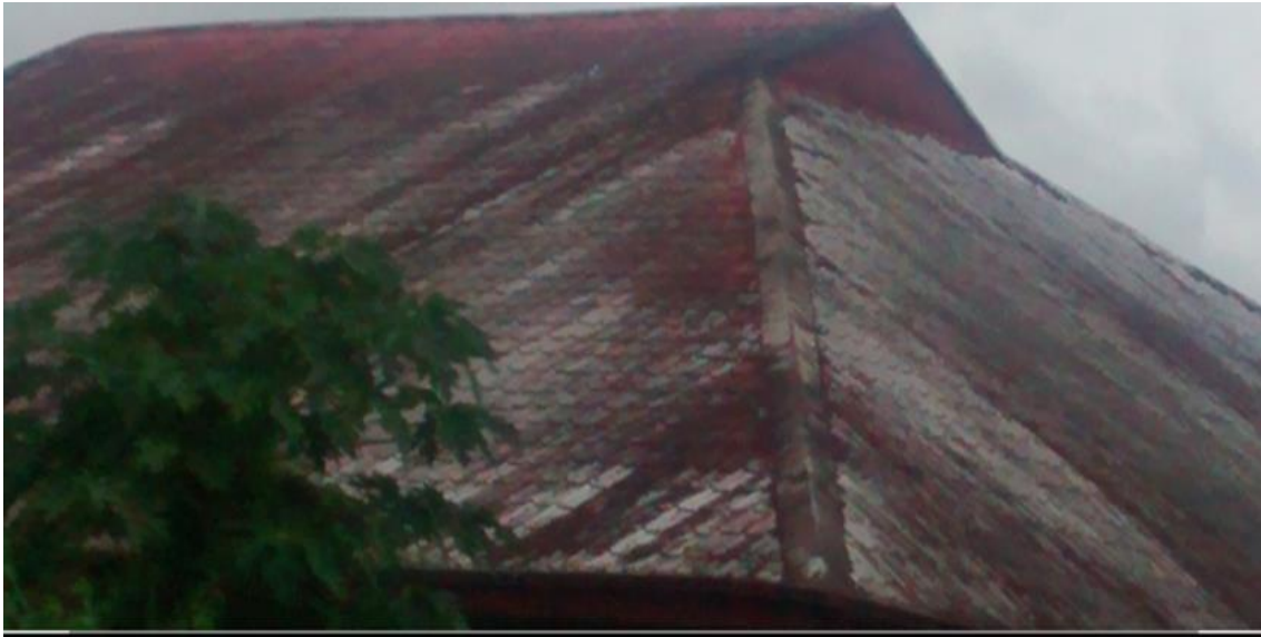
Figure 2.12 Discoloration of Aluminium Roofing Material Source: Field Work (2016)
