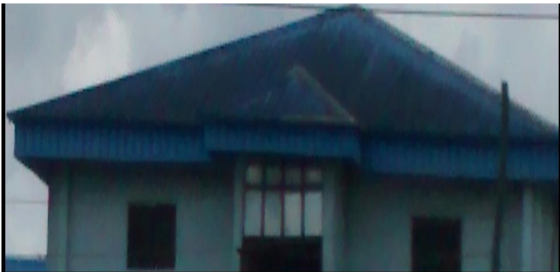
Figure 2.13 Blackening of Aluminium Roofing Sheet Source: Field Work (Pictured 2016)
