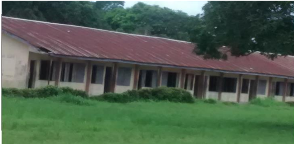
Figure 2.11 Corroded Roofing Materials Source: Field Work (2015)
