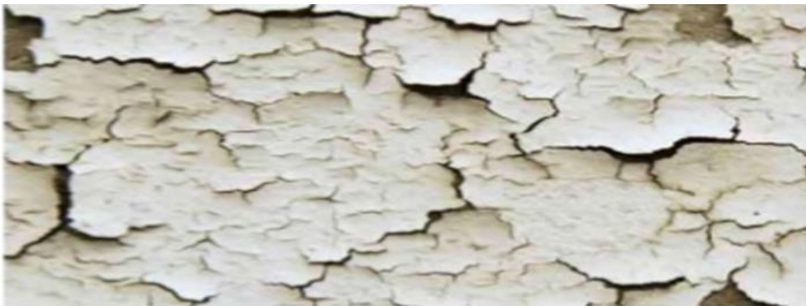
Figure 2.10 Deterioration (Flaking) of facade painting Source: Alaba (2014)
