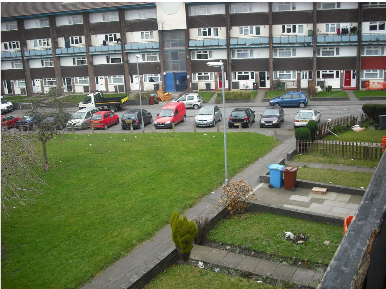
Figure 3 - The development before retrofit started.
