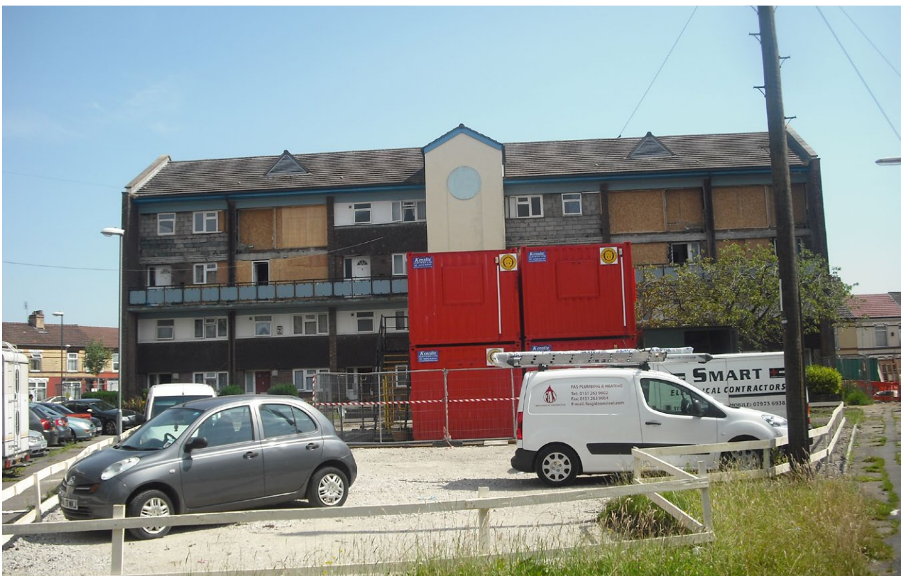
Figure 7 - The during the retrofit
