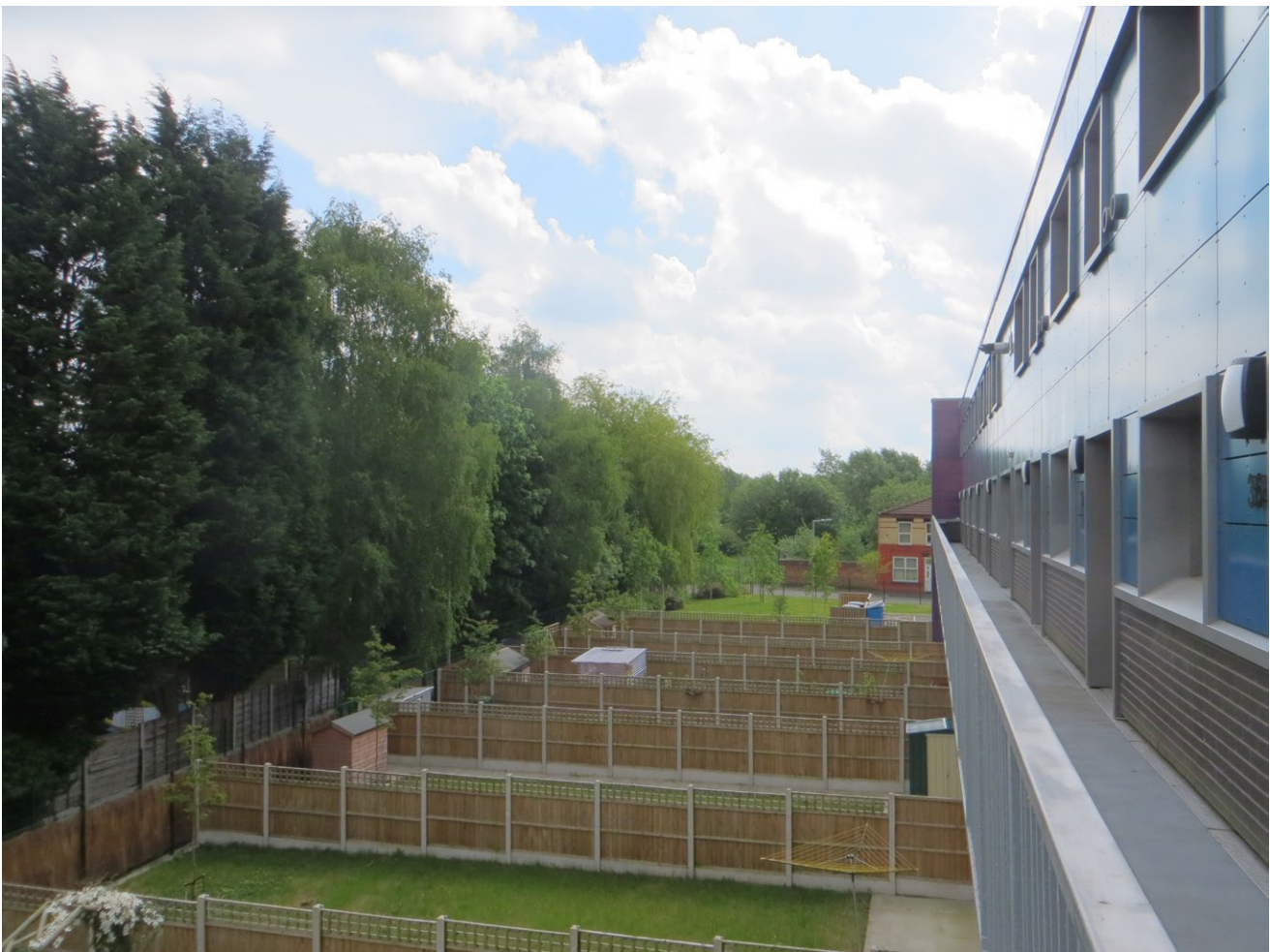
Figure 4 - View of tenants’ gardens
