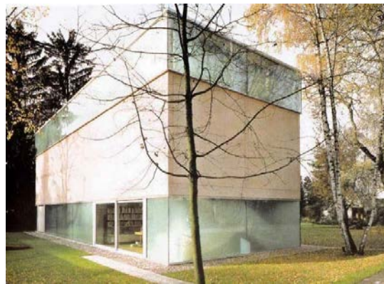
Figure 3.9 Integrated relationship between stone cladding and lightweight glass in Goetz Gallery, Munich. Herzog & de Meuron Archetektin (Hagan, 2001).
