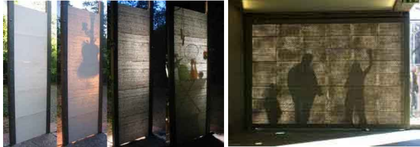
Figure 3.11 The use of translucent concrete as a design element in buildings (Litracon, 2017).
