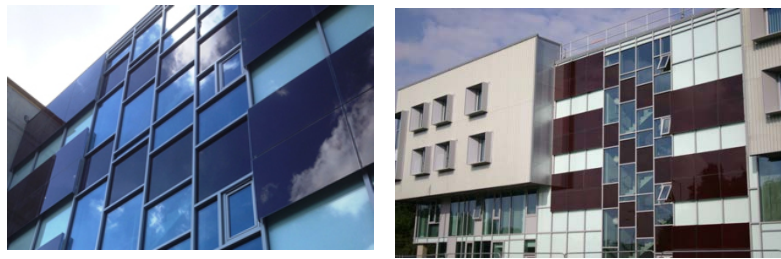
Figure 3.16 Future Business Center Cambridge with an integrated design pattern of opaque and transparent Photovoltaics (Polysolar, 2014).
