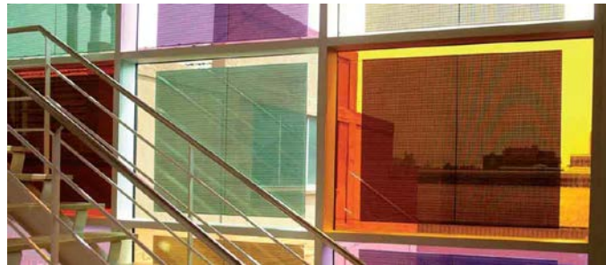
Figure 3.19 Semi-transparent BIPV façade Schott Iberica, Barcelona (SolarServer, 2015).
