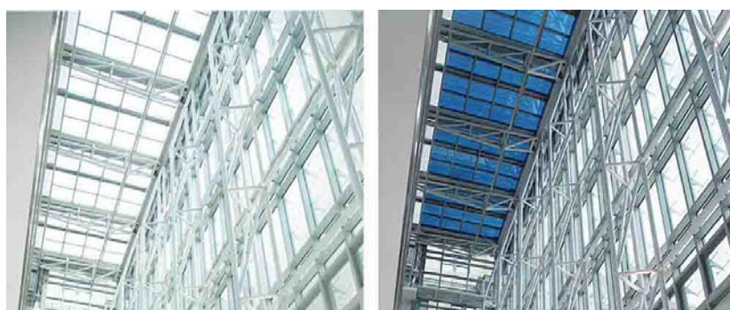
Figure 3.29 Dynamic glazing in the clear and opaque state (SageGlass, 2016a).
