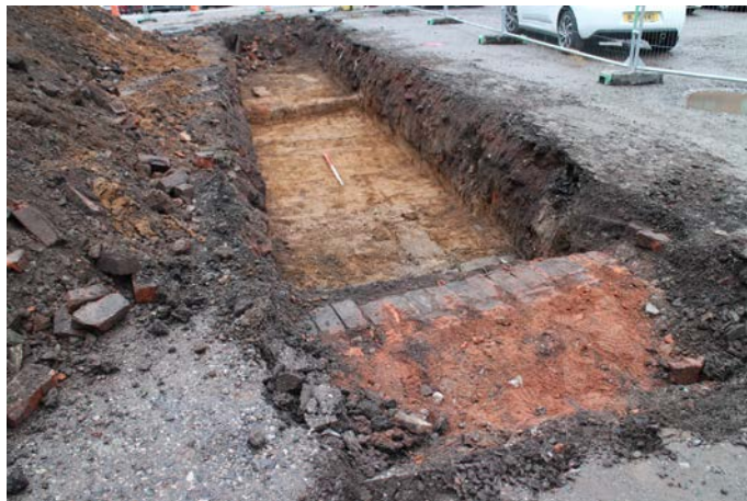
Plate 14: Trench 5 general shot, looking north
