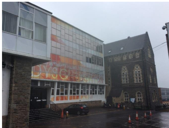
Figure 10: Current, Front Elevation of the George Thompson Building of University of Wales Trinity St. David (UWTSD)
