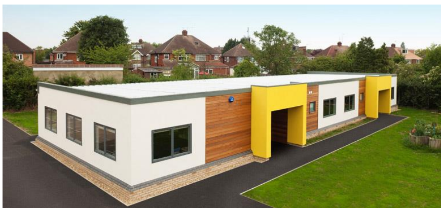
Figure 4: Permanent Modular Building – aesthetically less pleasant (Wernick, 2017d)
