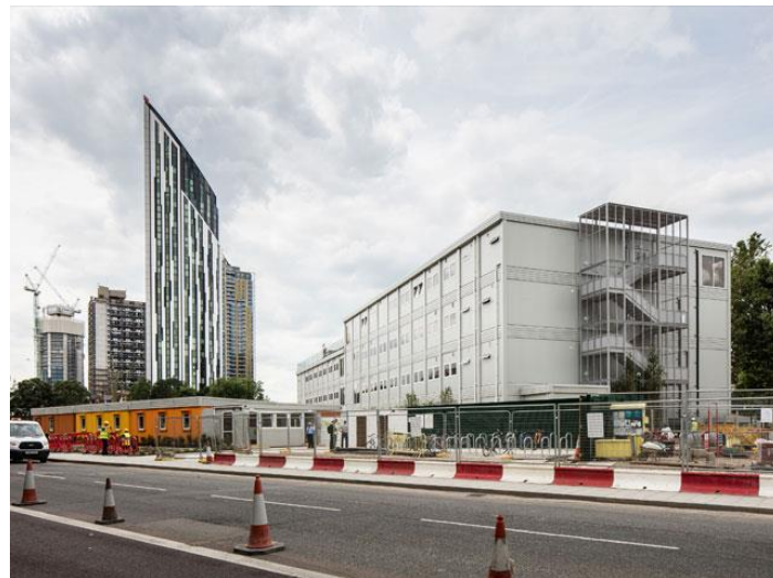
Figure 3: Temporary Modular Building – aesthetically pleasant (Wernick, 2017b)
