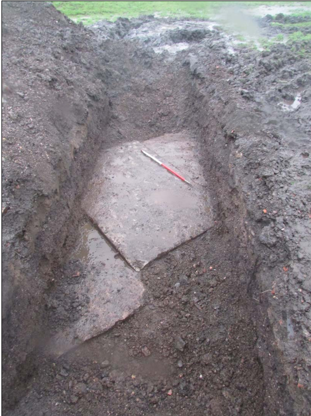
Figure 15: T2 looking east across the stone culvert.
