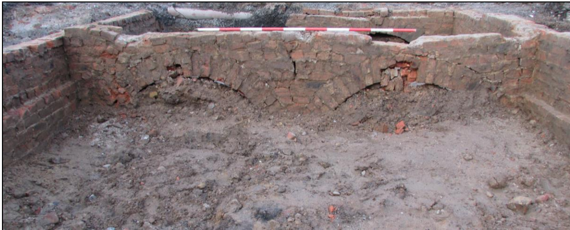
Fig. 19 Wall (181) was relatively intact but badly cracked in places, suggesting it may have been affected by subsidence.
