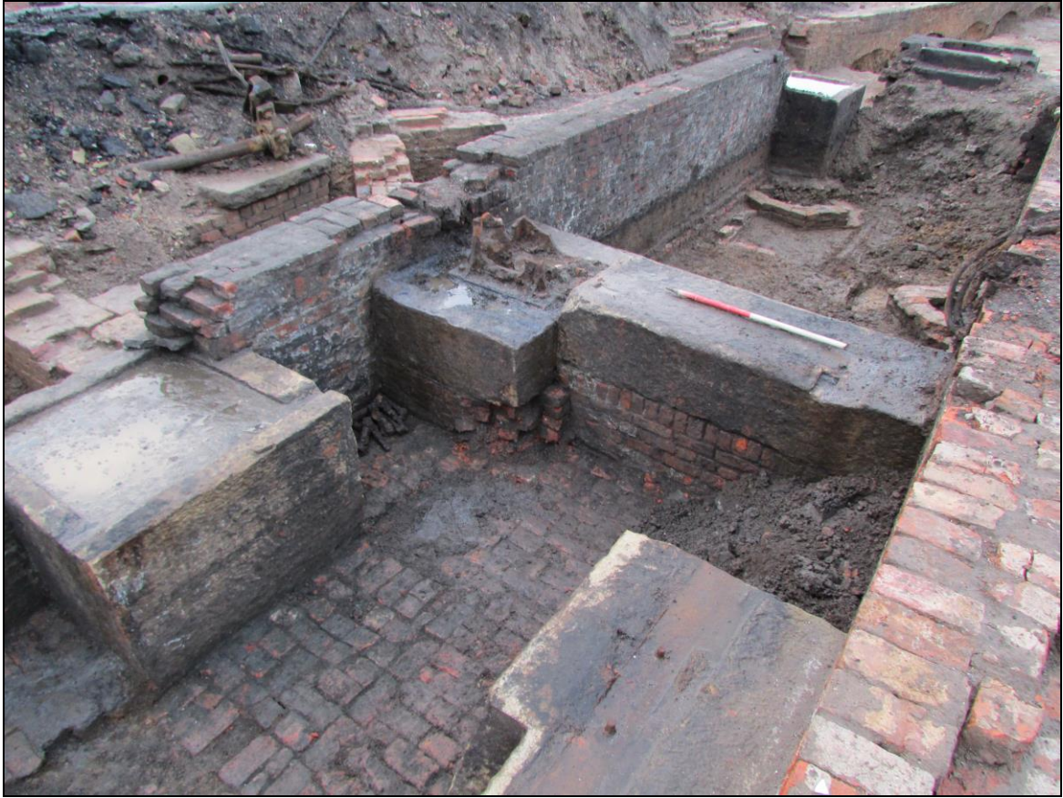
Fig. 48 The hydraulics for the capstans ran along this stone block (with the ranging rod). Note the driveshaft related to it located within the top left of the picture.
