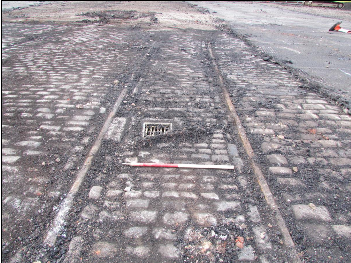
Fig. 38 An example of the cobbled surface and railway line belonging to the Railway Goods Yard.
