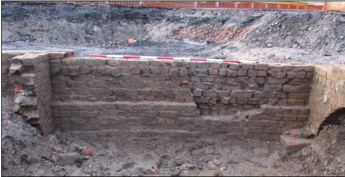
Fig. 16 Wall (085) with later repair, shown on the right.
