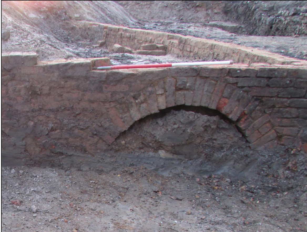
Fig. 13 Wall (032) showing the alternating header/stretcher construction of the archway.
