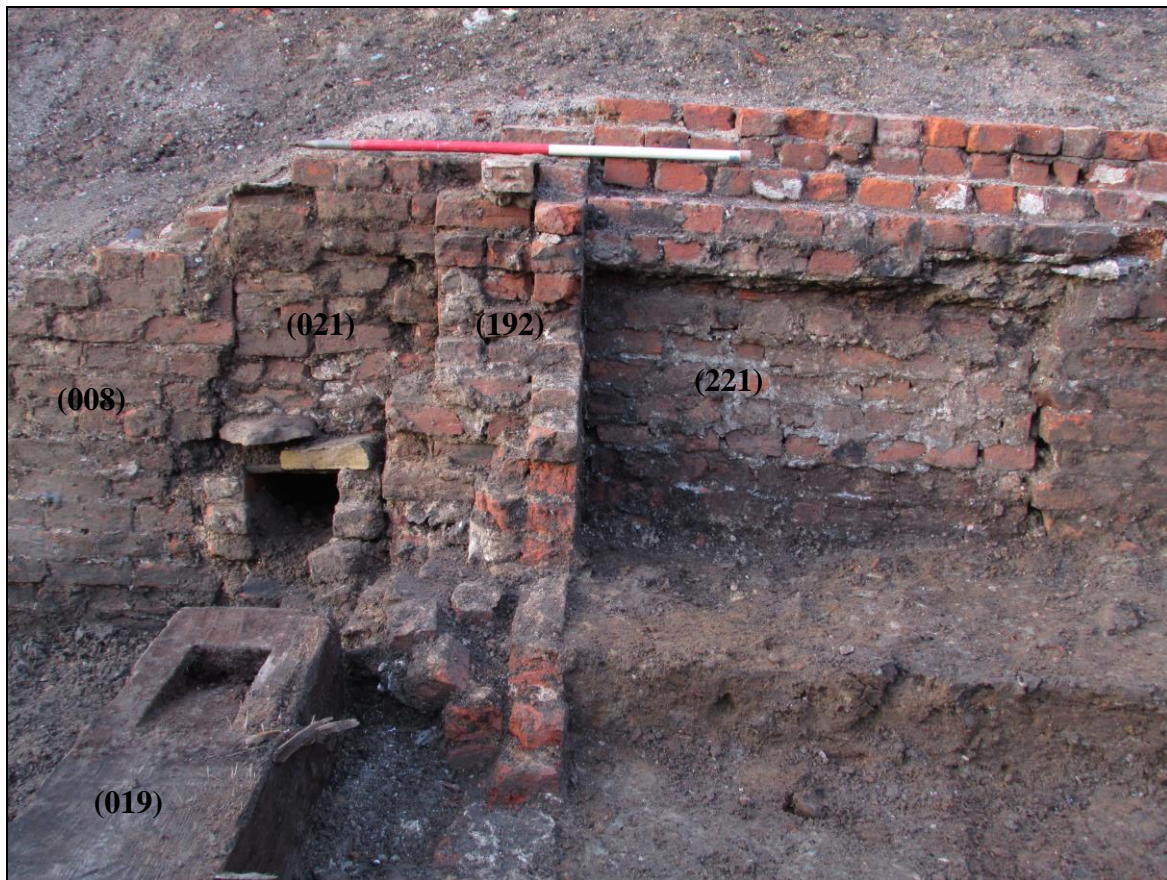
Fig. 20 The differing mortar between (008) and (221) shows where the Hospital Wing was added.
