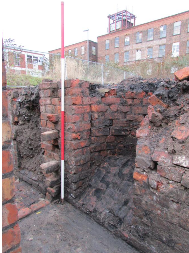
Figure 29, showing (041) a possible coal chute.
