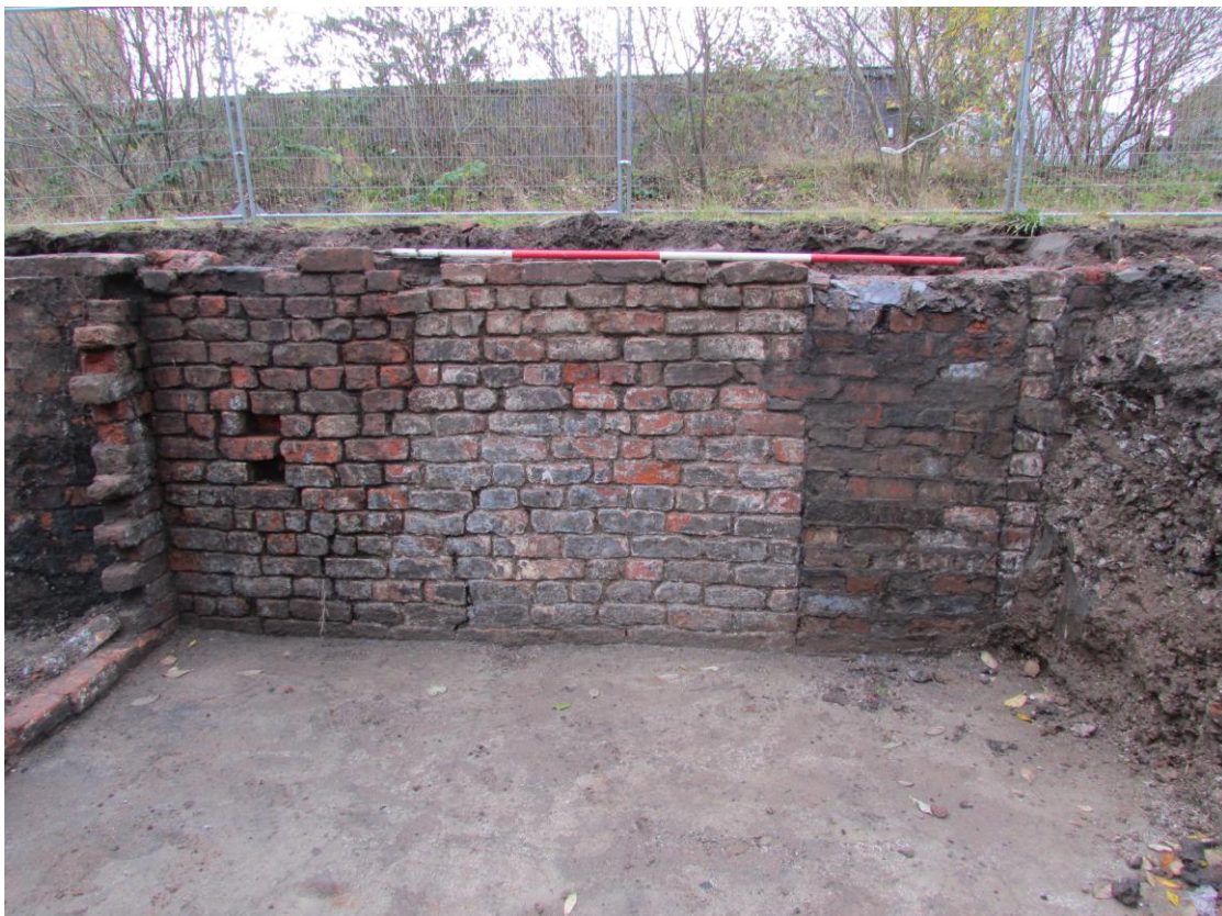
Figure 41, South wall of Cellar 1, to the right of the photograph it is possible to see the blocked doorway.
