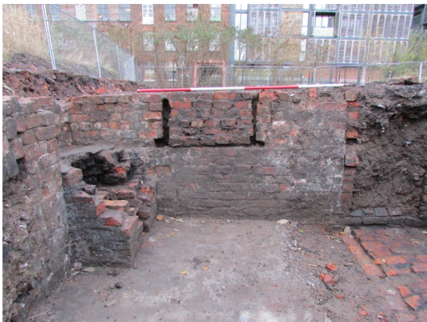
Figure 32, showing the internal detail of (031) the possible blocked light in Cellar 1, with (034) to the left of the picture.
