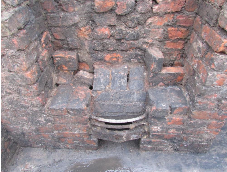
Figure 27, showing a close up detail of the fireplace in Cellar 2.
