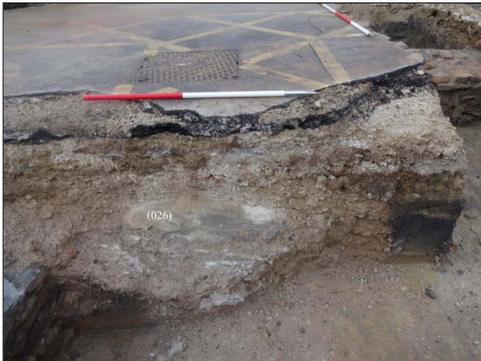
Fig 17: The eastern end of T2 looking north, with [032], the intrusion and disturbance of the archaeology of the manhole inspection chamber and associated concrete surrounding (026).
