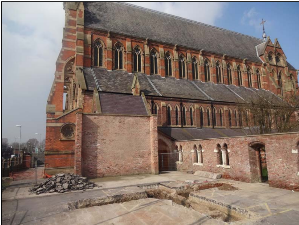
Figure 1: Gorton Monastery with the cloister garden perimeter wall located on the right.
