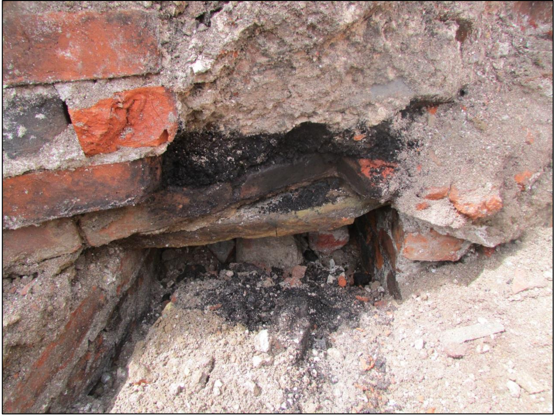
Fig. 8 Close up of possible flue, with in situ heat affected bricks and black ashy deposit above. This was located approximately 1.50m below the ground surface
