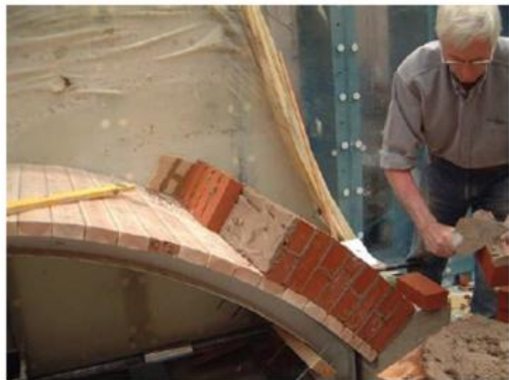
Figure 2.4: Header bonded arch barrel construction
