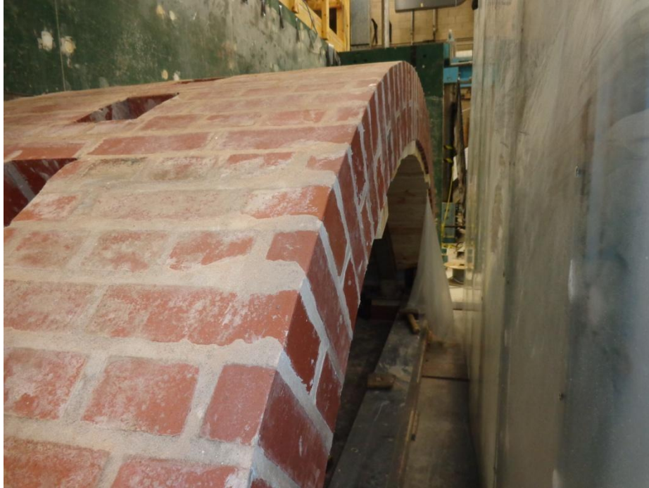
Figure 2.14 – Completed brickwork arch before fixing chamber wall into position
