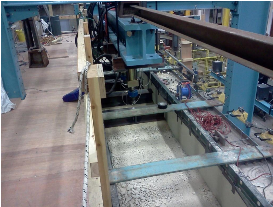
Figure 2.19 – Final Fill level, top level lateral ties visible, longitudinal reaction beam with actuators attached
