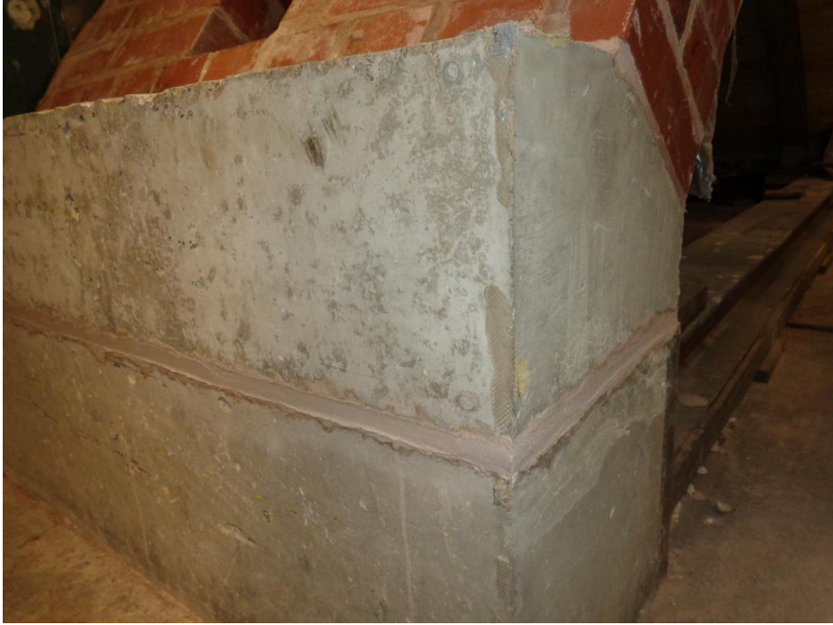
Figure 2.10 – Concrete abutments showing skewback with horizontal mortar joint and tie beam
