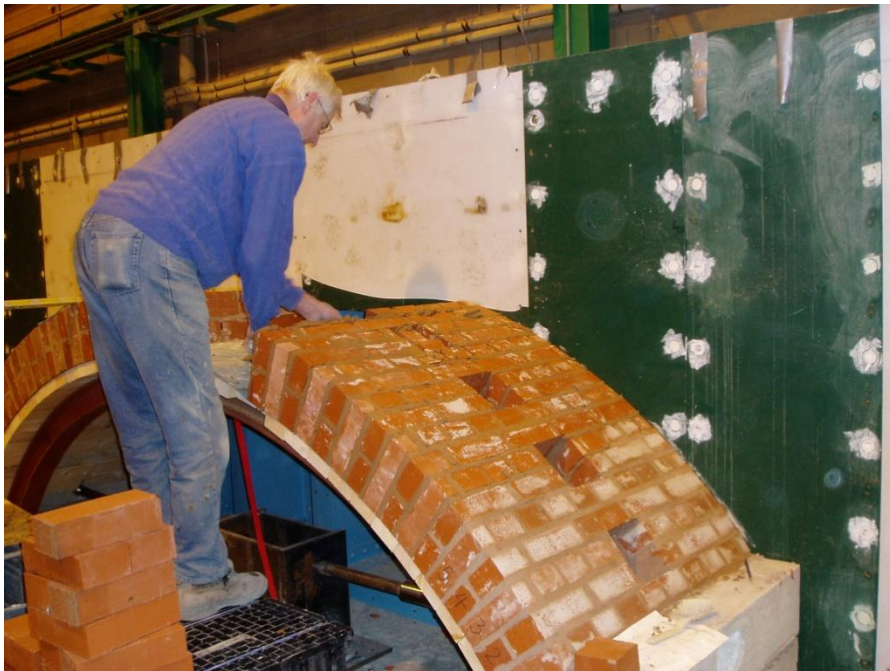
Figure 2.13 – Arch near completion with recesses to accommodate soil pressure cells
