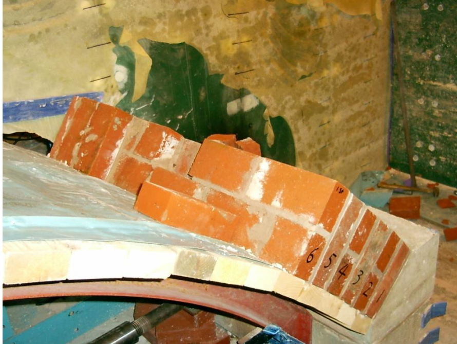
Figure 2.12 – Brickwork configuration and construction sequence
