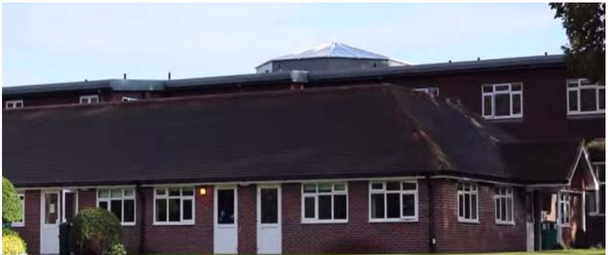
Figure 8.19 - Outside the building, with new atrium visible
