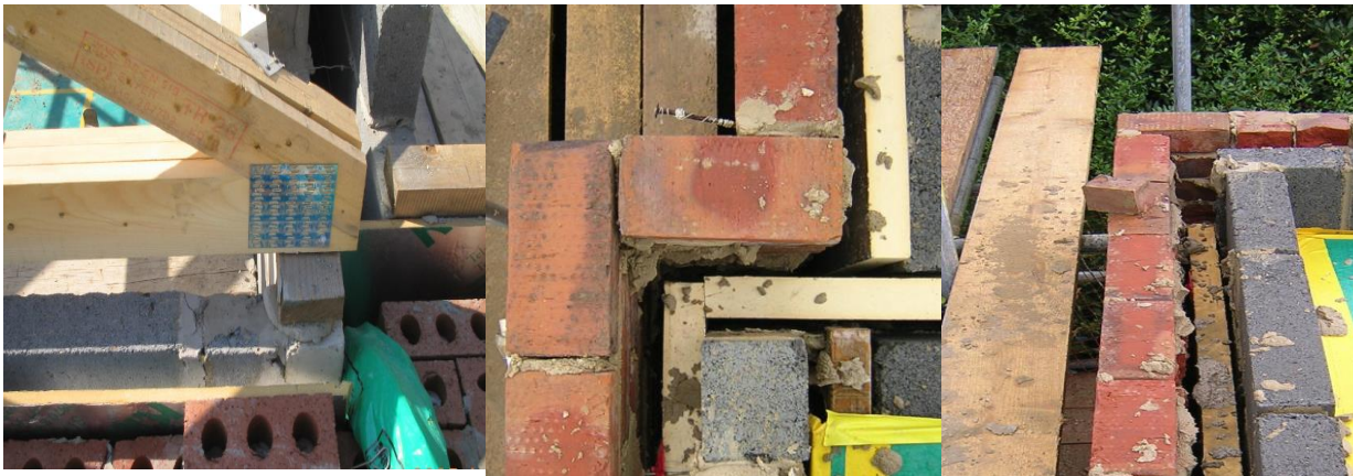
Figure 5. Poor workmanship, joints and debris making effective joints difficult (source Johnston et al 2011; Smith et al 2005)
