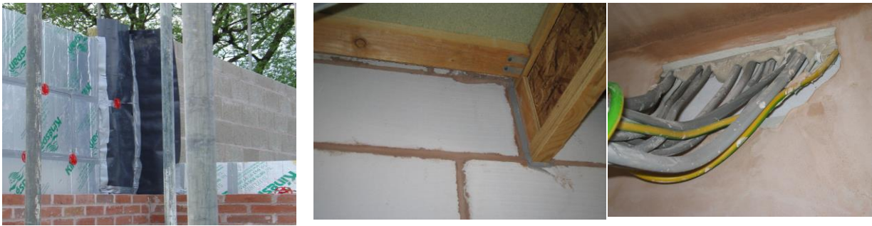
Figure 6. Examples of sealed masonry and good practice (source Johnston et al 2011)
