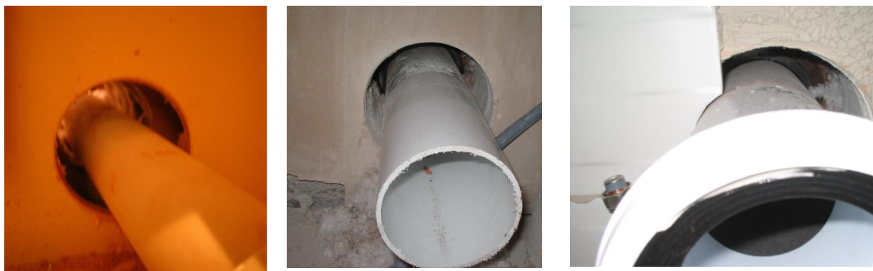
Figure 2. Service penetrations through fabric (source Johnston et al 2011)
