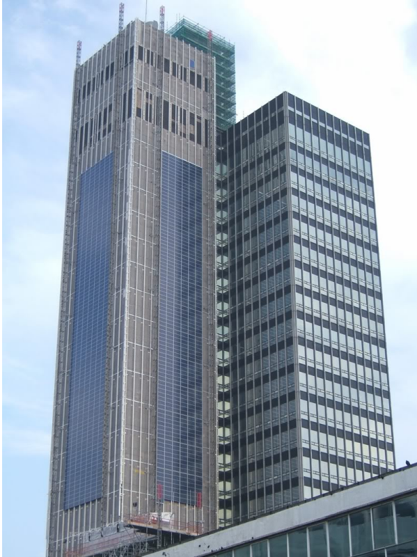
Figure 31 | The CIS service tower during intervention in 2005, when three of its four side were completely clad in PV panels; with the design team of Solarcentury working on this £5.5 million project, the CIS mega-scale refurbishment has resulted in the largest commercial solar façade in Europe.
