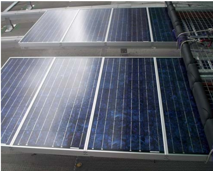
Figure 32 | The PV module chosen for the overcladding of the service tower. A total of 7244 80W photovoltaic cells cover the entire surface, and were manufactured by Sharp to Solarcentury’s design. (Credits: CIS. Source: http://www.solaripedia.com )
