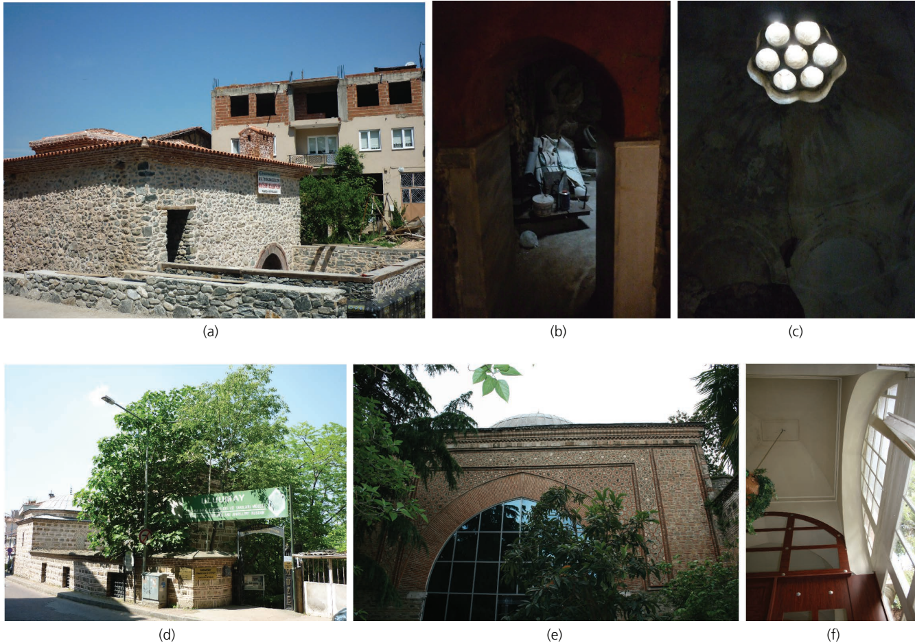
Figure 1. Demirçi bathhouse with internal views of the hamman showing the top-lit dome of the studied northern hot room ((a)-(c)), Uluymay Museum (d) and Muradiye Madrasa ((e) and (f))
